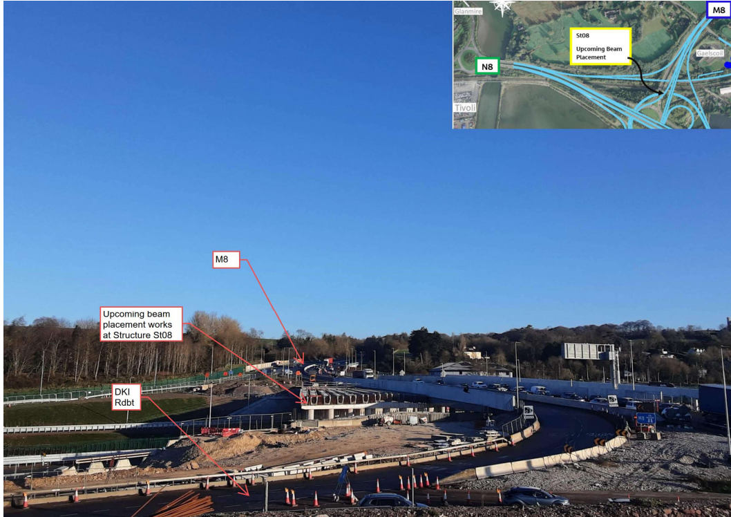
Upcoming beam placement at Structure, ST08.
