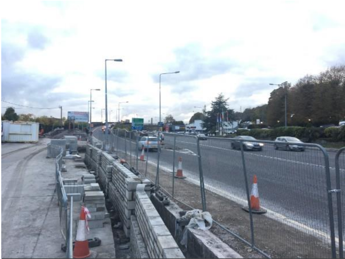
Boundary wall under construction at Silversprings, facilitating road widening
