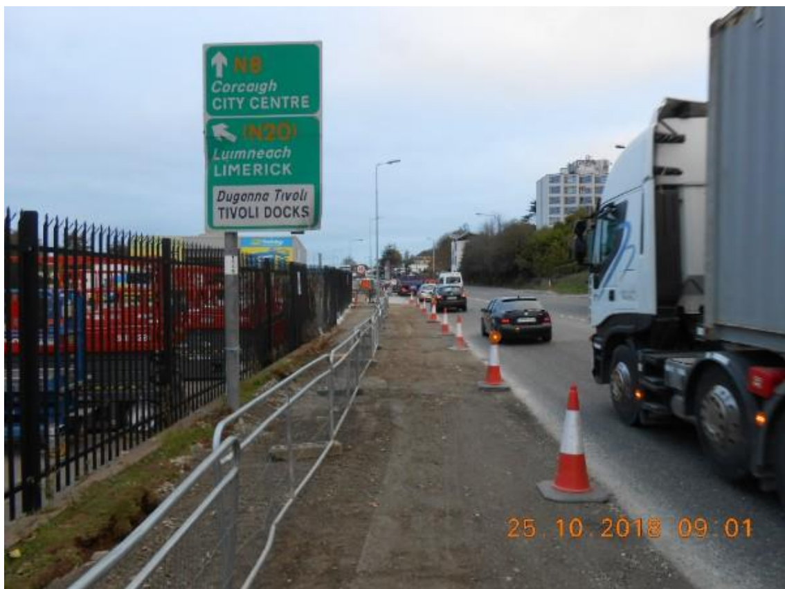
Road widening works at Silversprings ongoing
