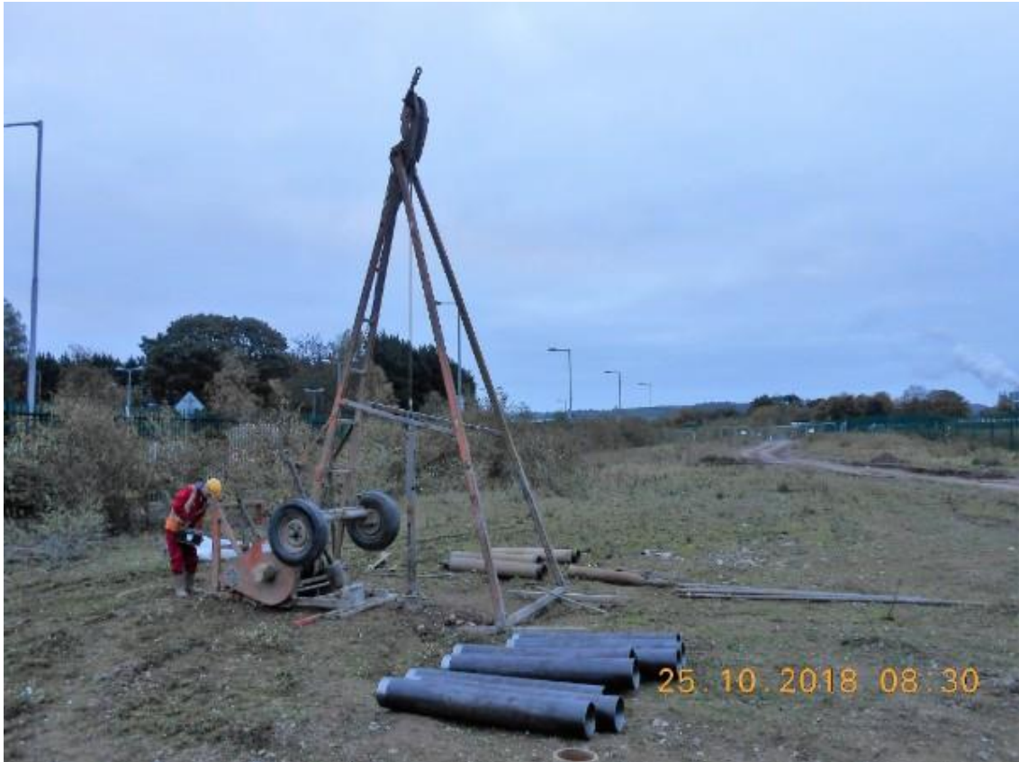
Ground Investigation Works south of the N25
