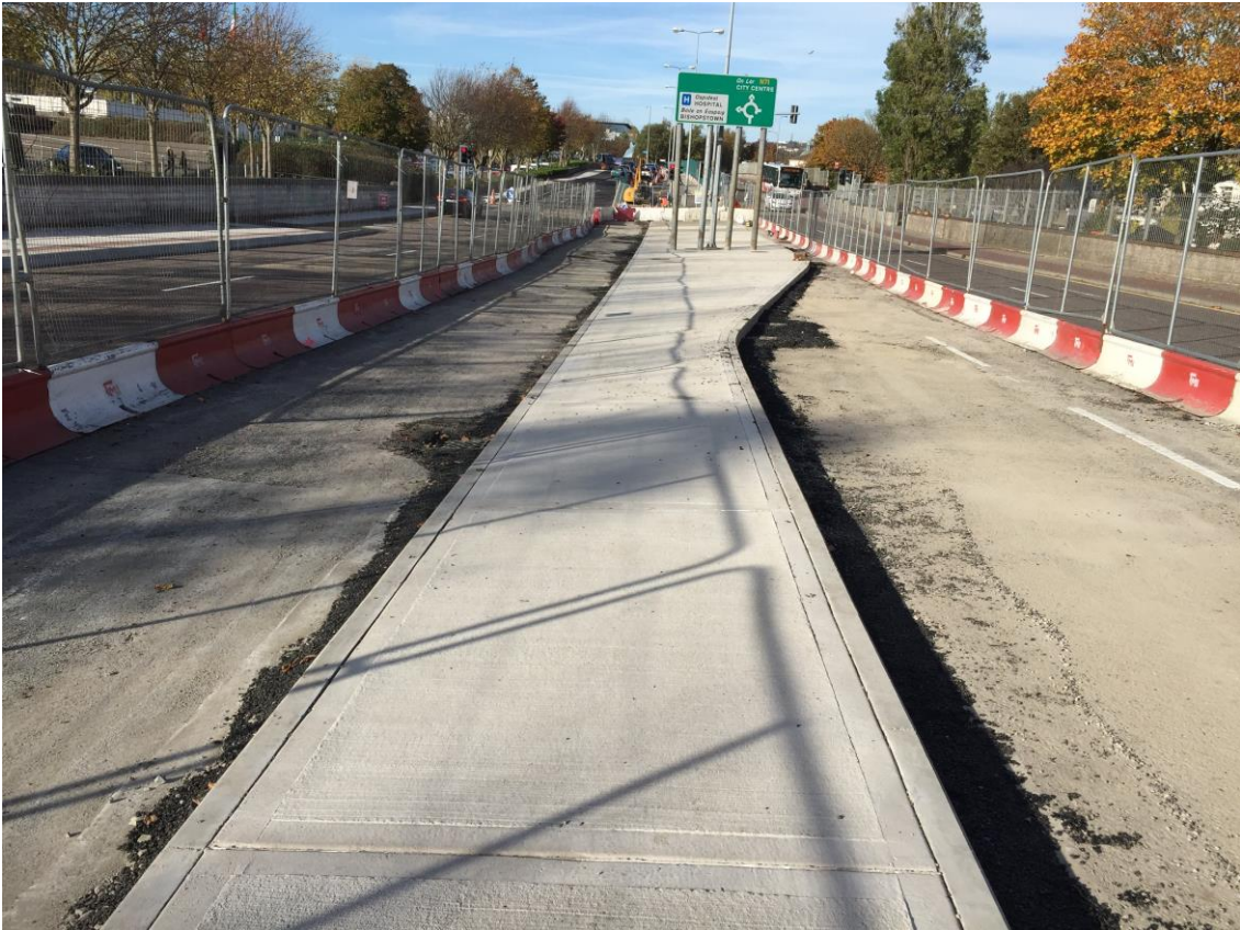
Sarsfield Road median works looking north
