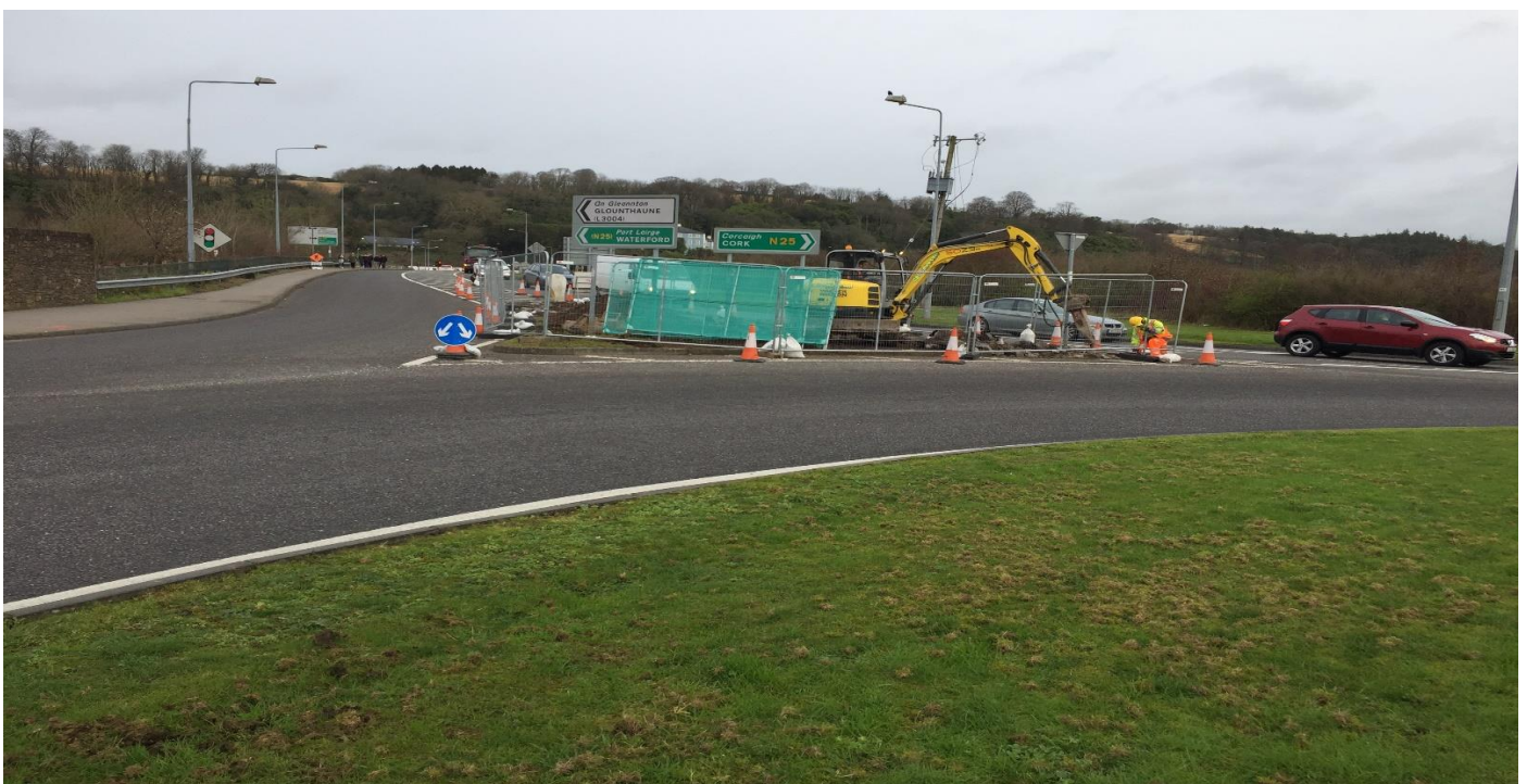
Removal of traffic island north of An Crompan Roundabout
