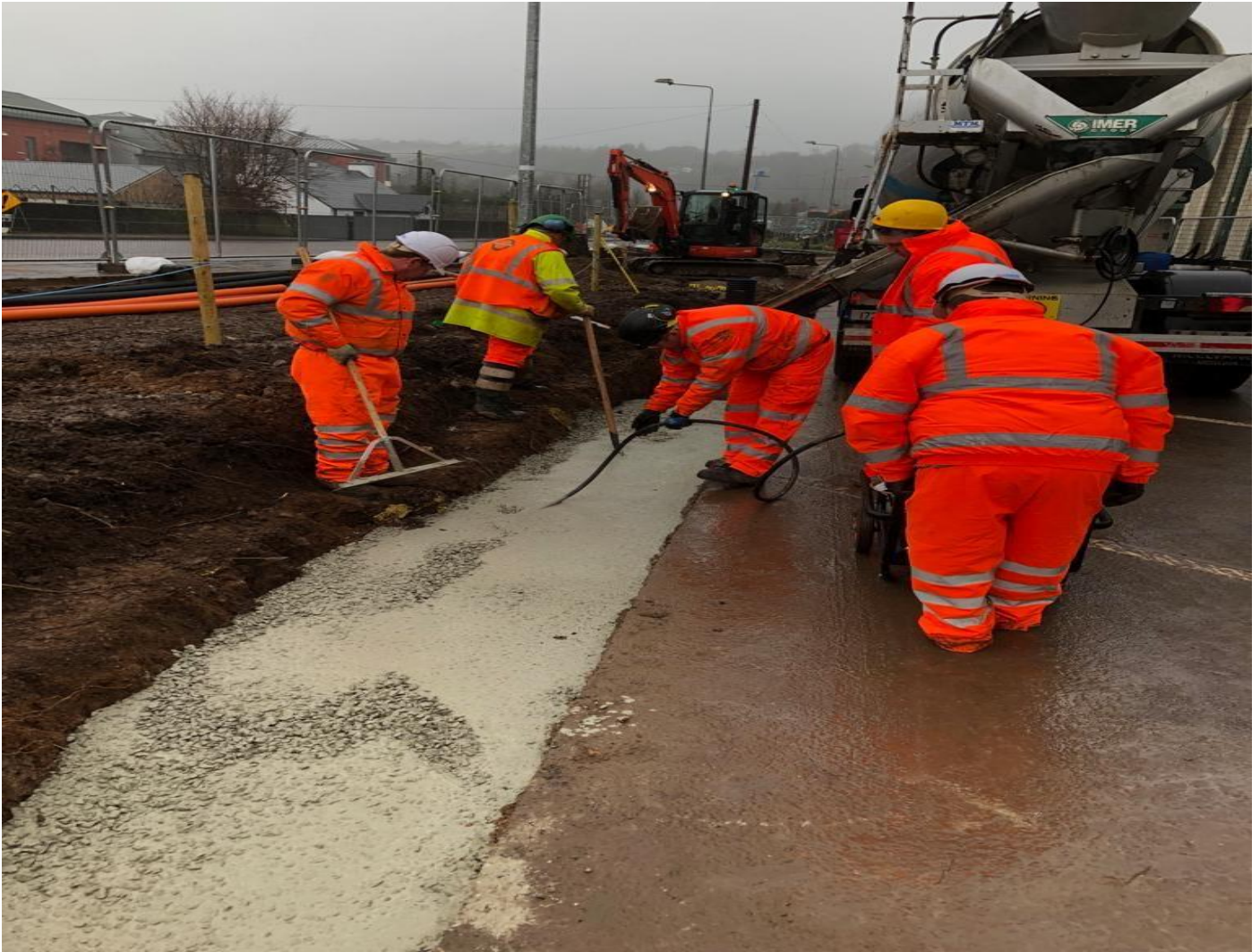
Concrete foundation being poured for new boundary wall at Jones Engineering building
