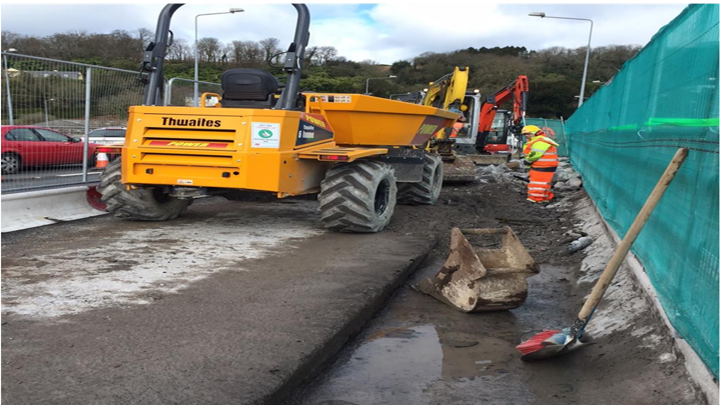
Bridge deck exposed at eastern section
