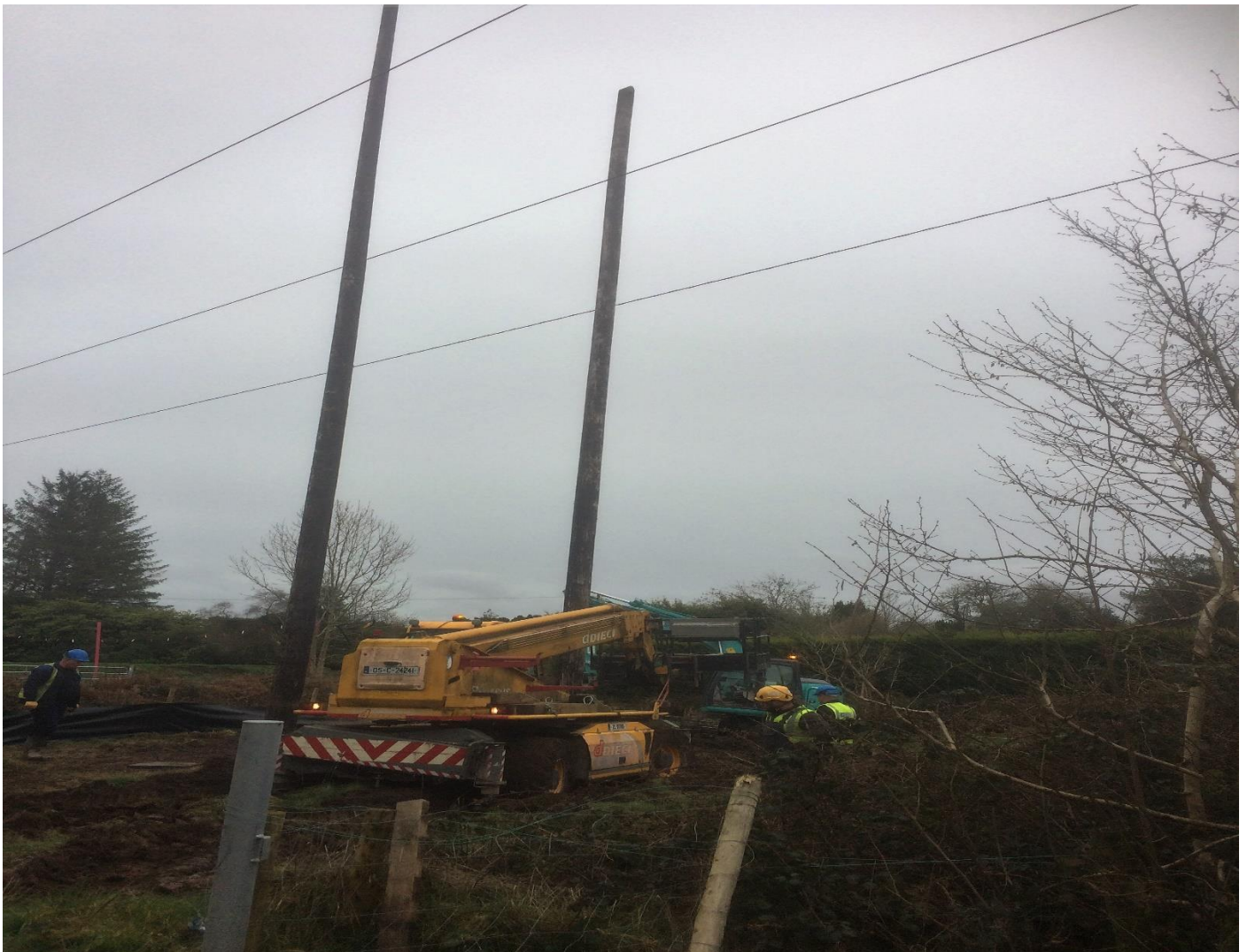
ESB crews erecting new pole set North of Ballyvourney/Macroom
