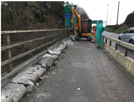
Dunkettle Interchange Upgrade: Parapet upgrade works and cycleway/ pedestrian walkway getting underway
