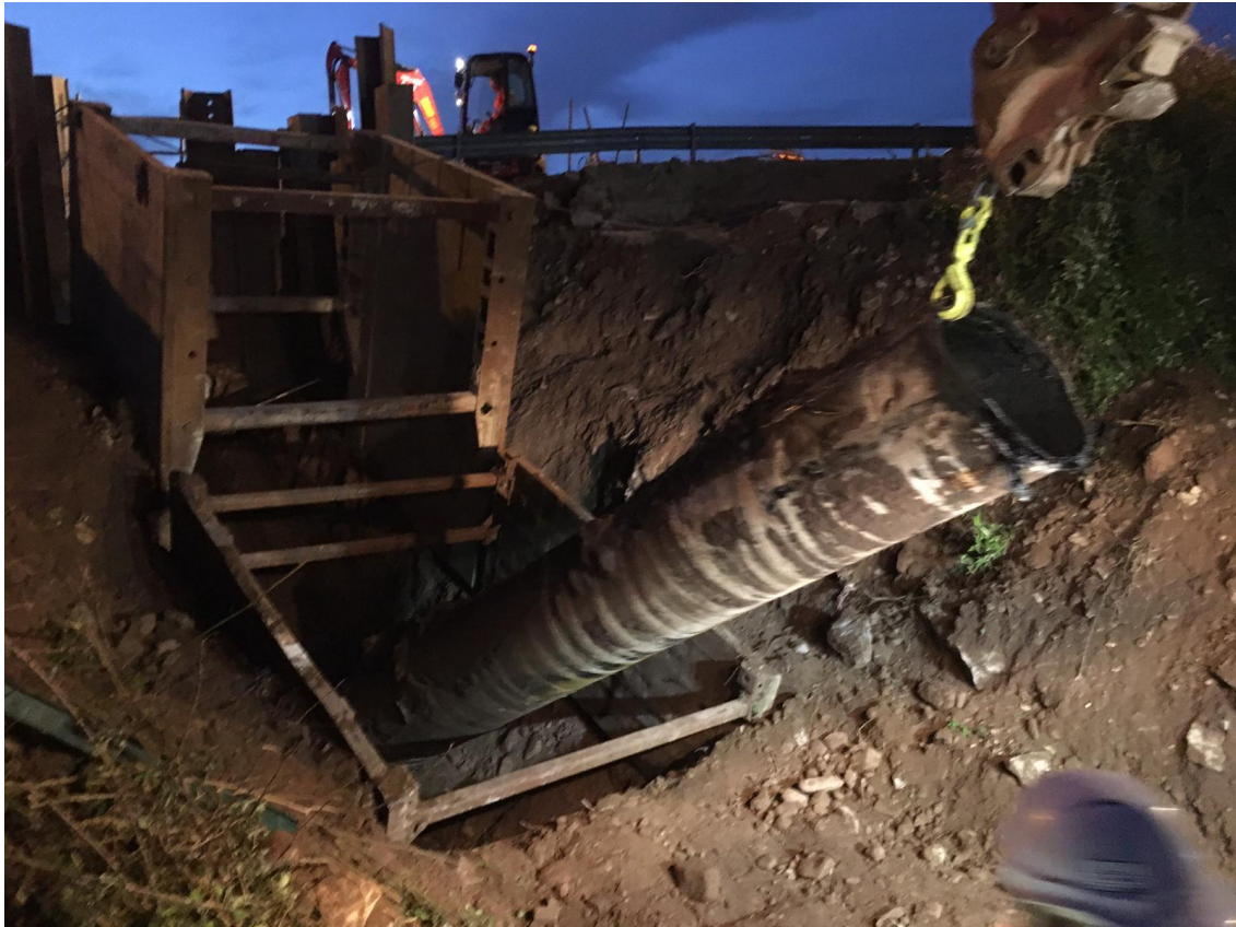
Section of the old watermain being removed in the early hours of Saturday 30 th May 2020.
