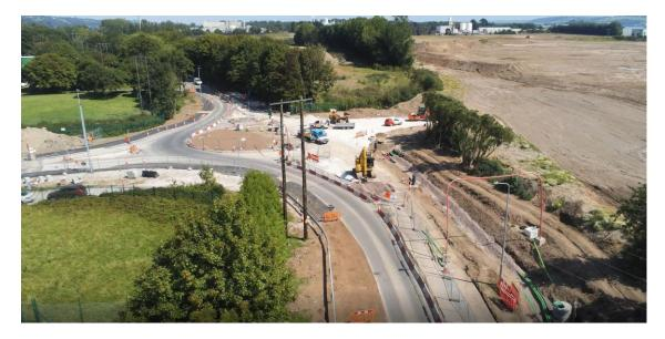
Preparatory works for surfacing on the southern section of the new R623 roundabout nearing completion
