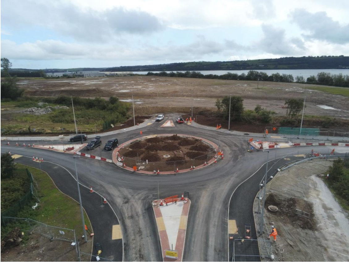
View of the surfacing works completed at the new R623 roundabout
