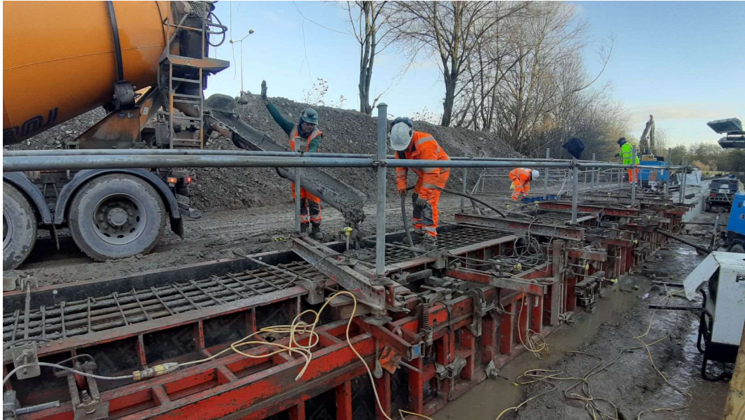
Concrete being poured to form the support beam for the concrete protection slabs at the gas transmission main site
