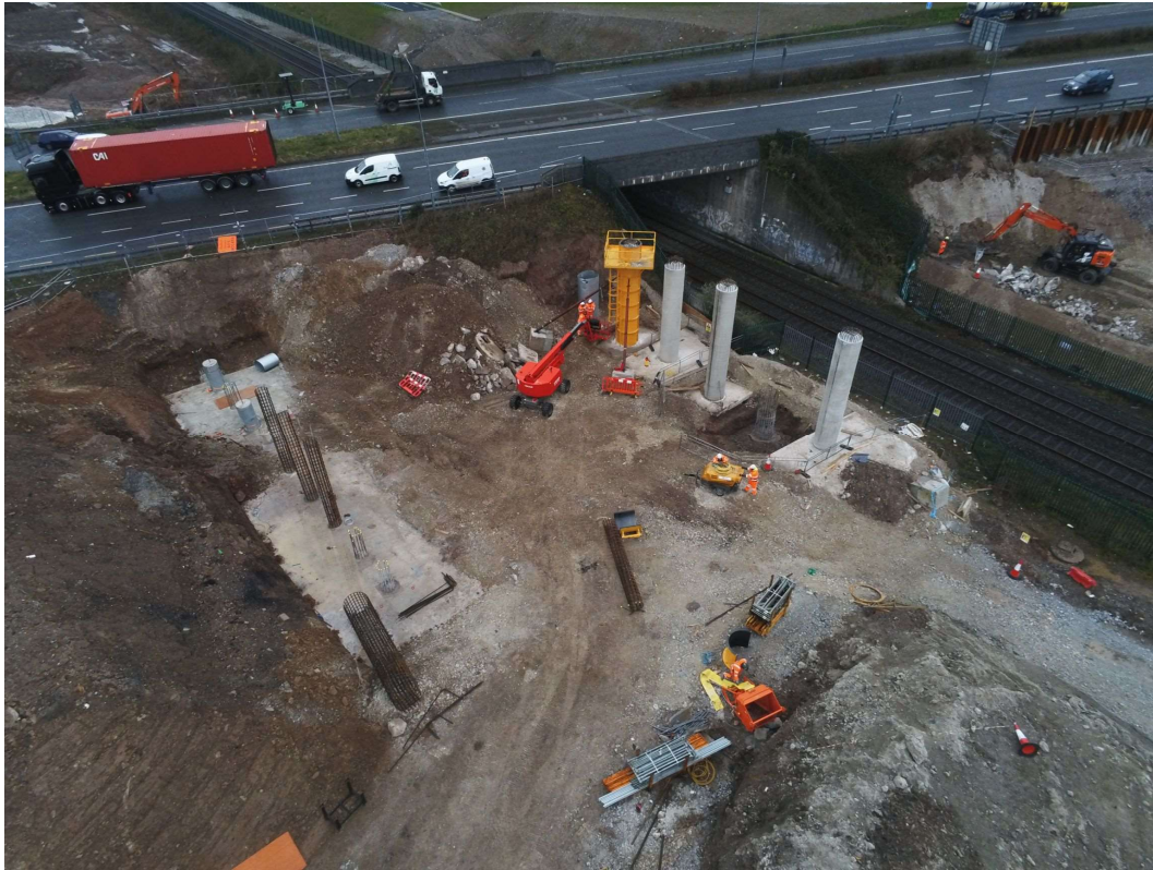
Aerial shot of column construction works in the area south of the Cork-Midleton railway line, immediately east of the existing N8 Cork/Dublin Motorway
