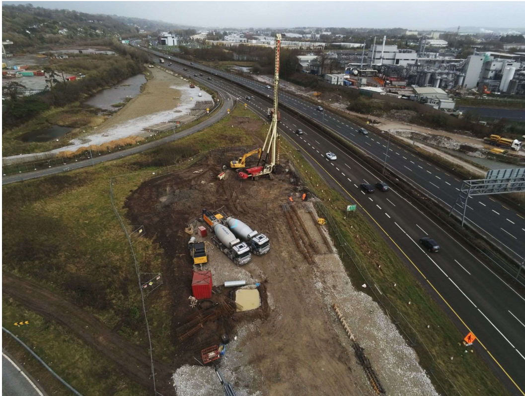
Piling works advancing at the northern abutment of what will become Structure ST01
