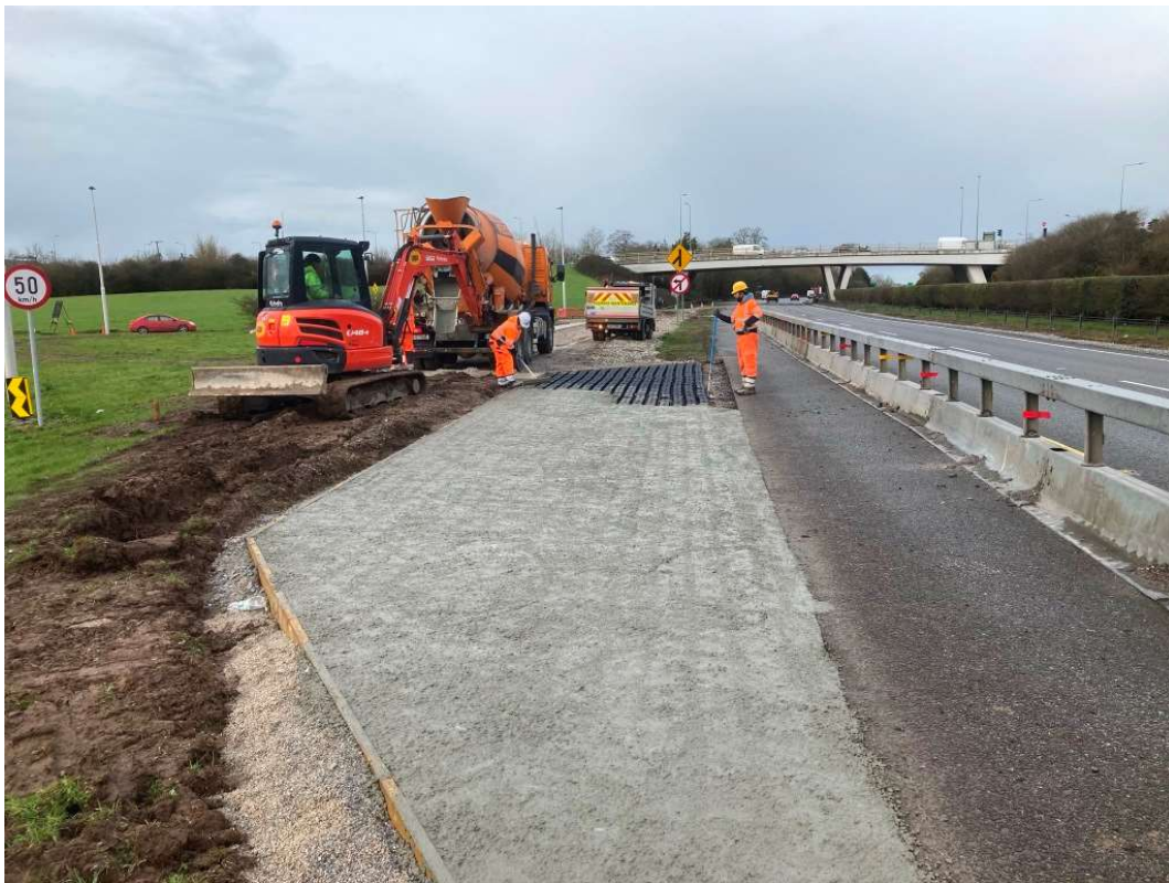
Construction of a lay-by advancing at Little Island Interchange
