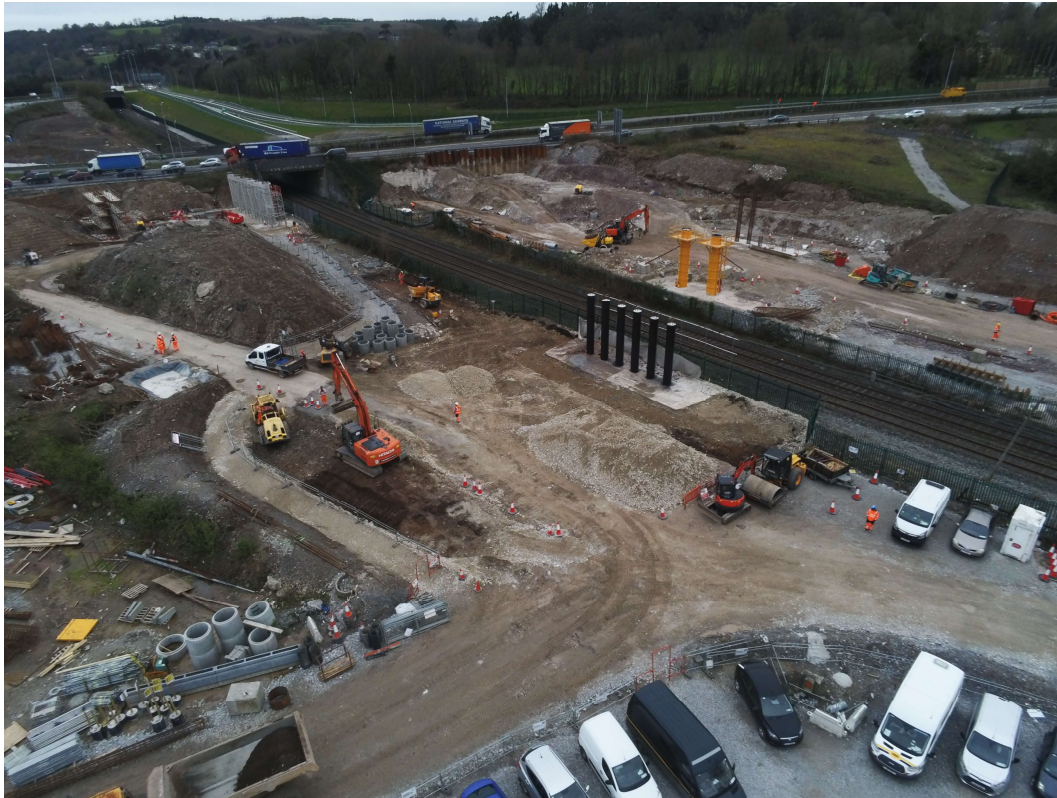
Progress photograph showing column construction on both of the two new rail crossing bridges in the area east of the existing M8
