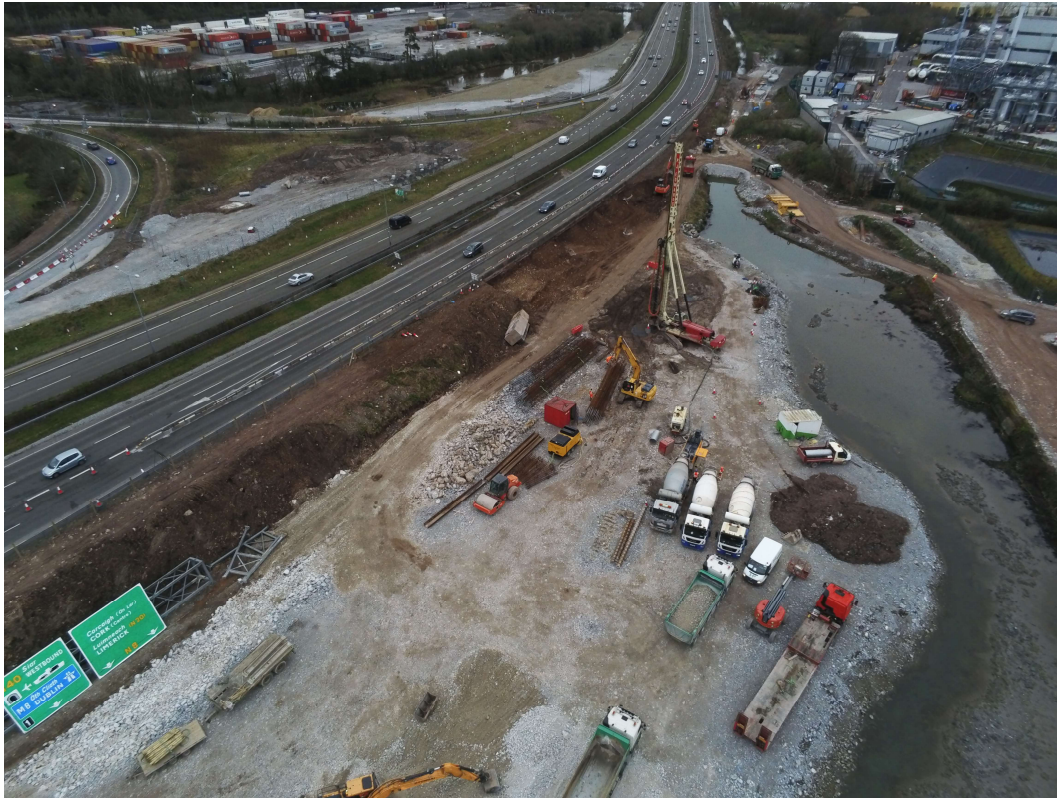
Piling works underway on what will become the southern abutment of the new N25 bridge crossing, east of the existing Dunkettle Interchange
