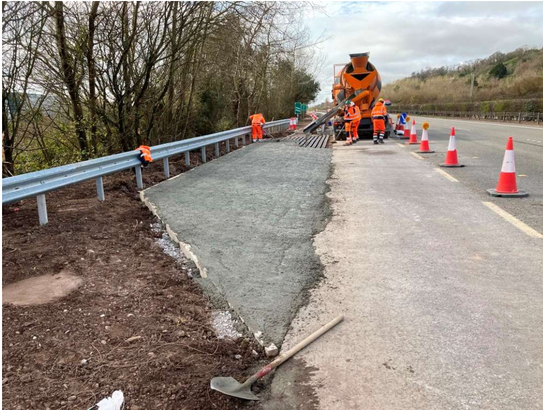
Concreting works ongoing in the lay-by area in the new ITS site west of Little Island Interchange adjoining the N25 westbound lanes
