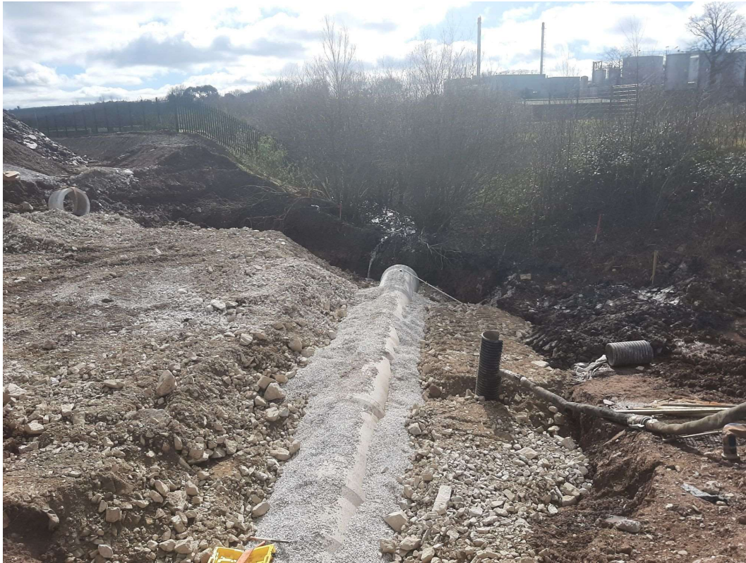
Culvert installation works nearing completion as part of overall road drainage arrangements on proposed Link Q
