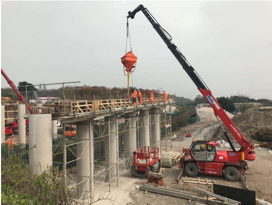
Concrete works being completed for the crosshead of Structure ST08 parallel to the M8 Southbound.
