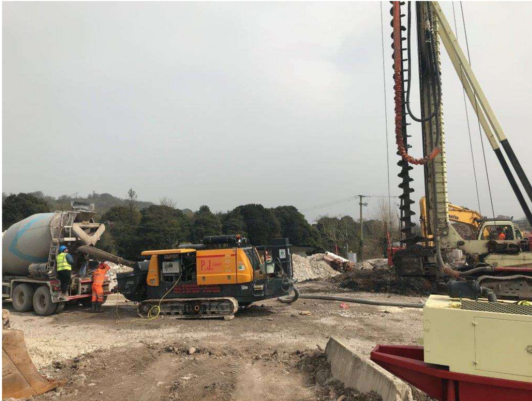
Piling works being undertaken using the Continuous Flight Auger (CFA) method
