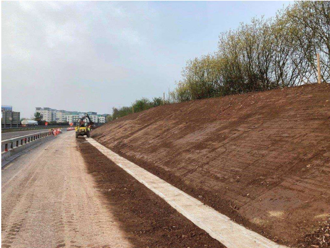
Topsoiling works being completed on the N40 Eastbound
