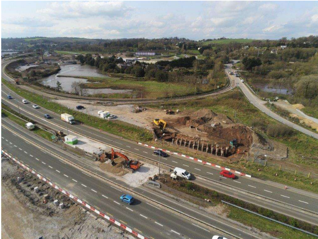
Preparatory works for the piling works in the N25 central median being undertaken.
