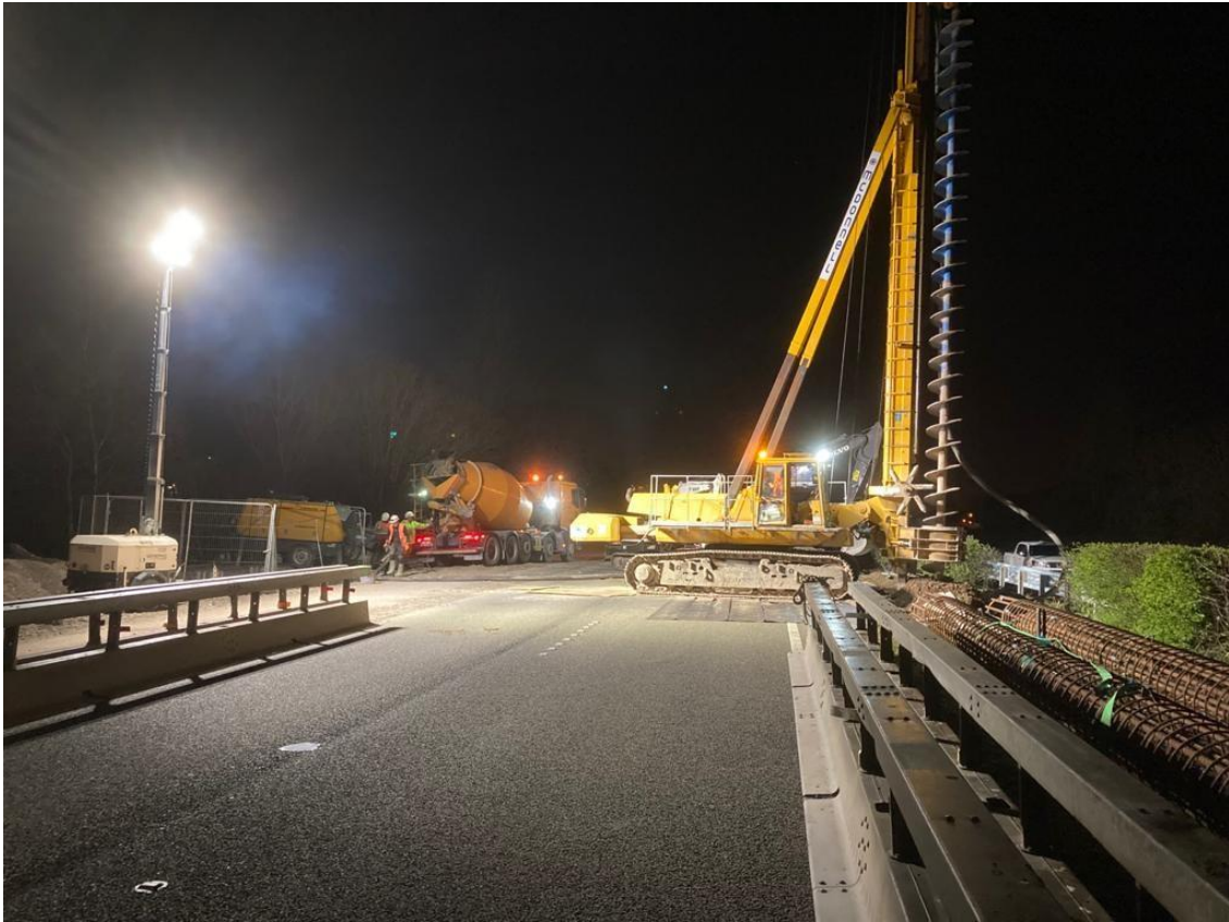
Bored Piles being installed in the central median of the N25 under a night time closure.
