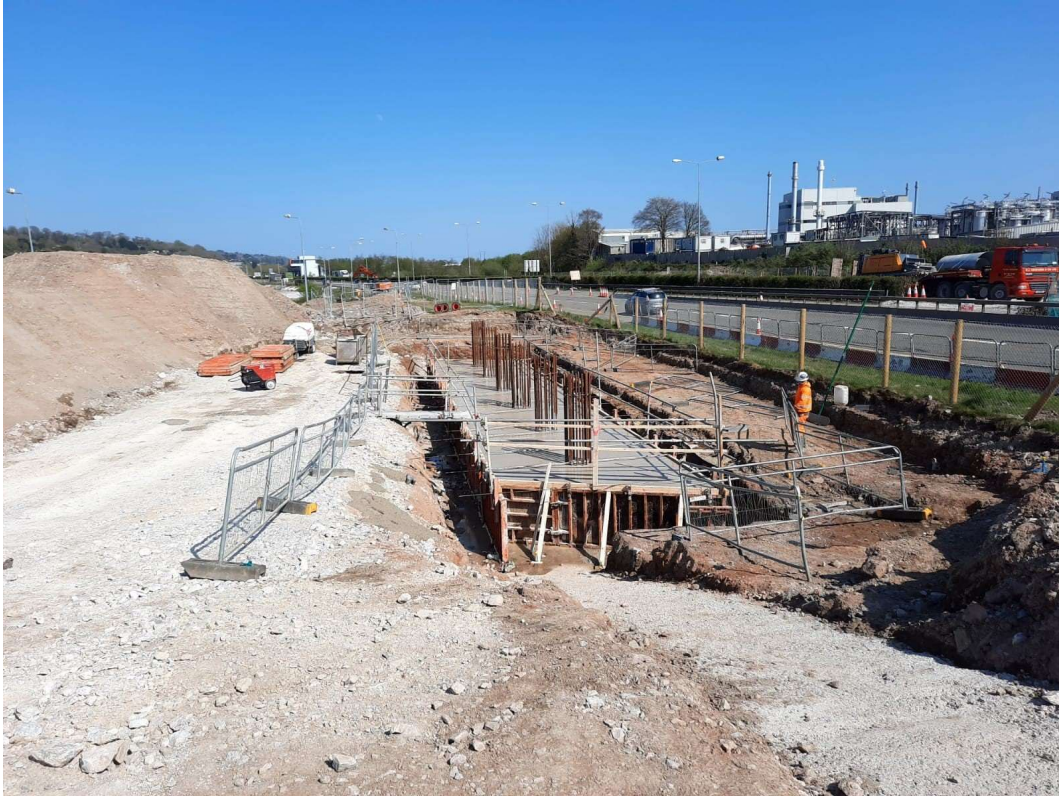
Completion of the pile cap for the ST01 northern abutment
