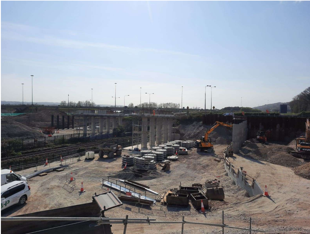
ST08 northern abutment being progressed parallel to the M8 southbound
