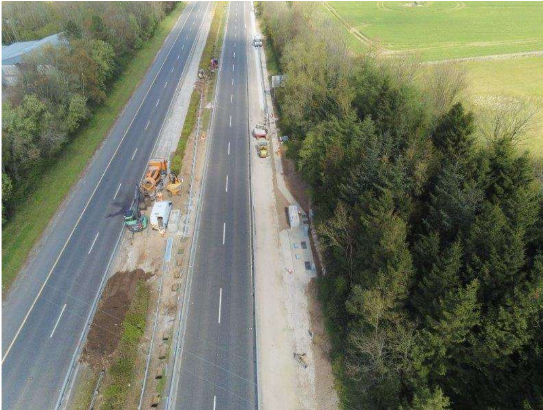
Safety barrier installation ongoing on the M8 southbound
