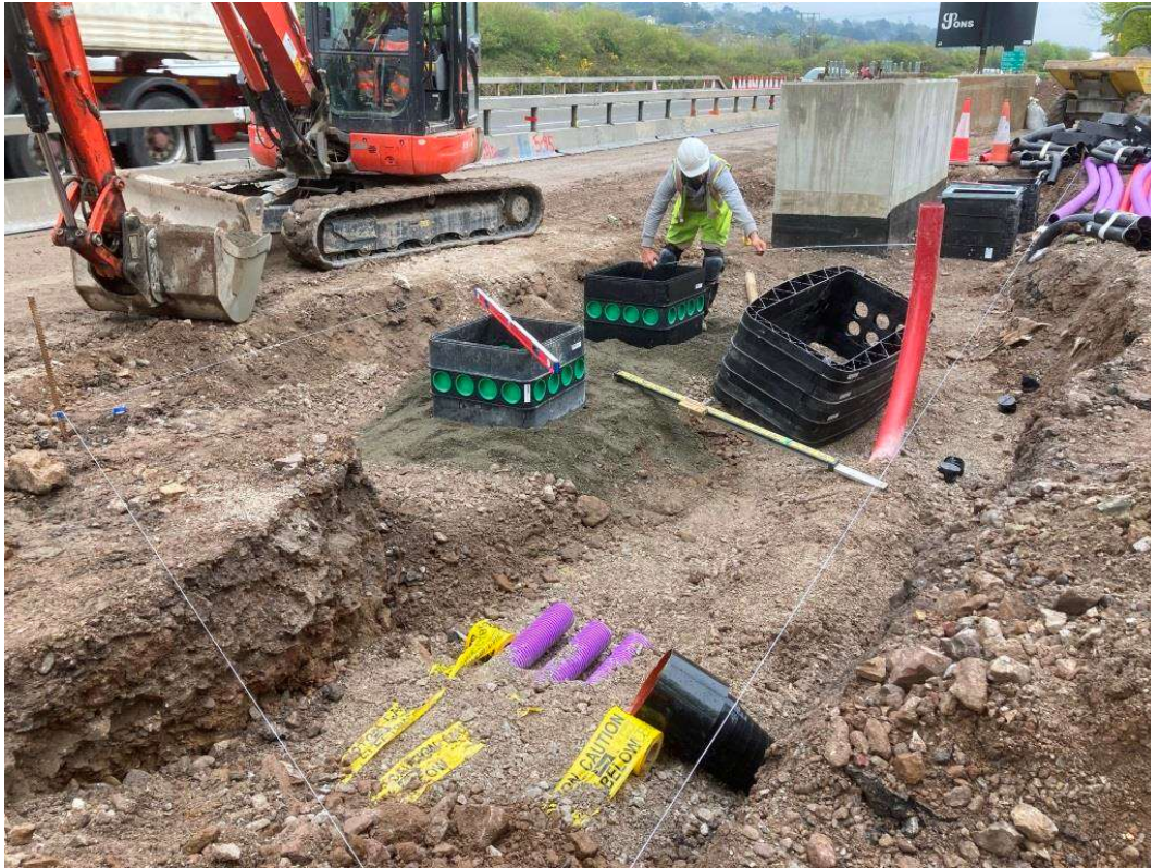
Ducting chambers being prepared on the N25 westbound southern verge
