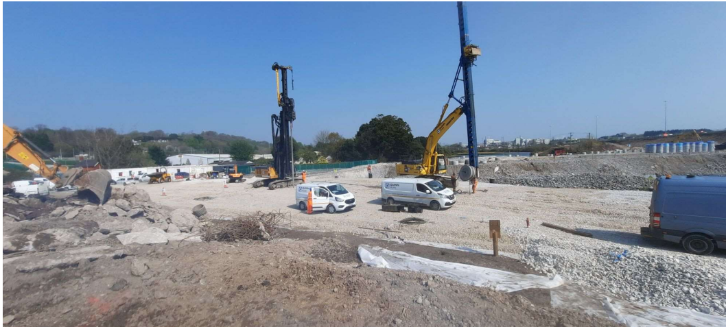
Vertical drain installation works ongoing on Link F north west of the Dunkettle Interchange Roundabout.
