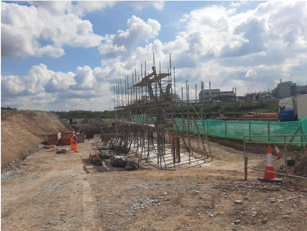
Preparation for the installation of the columns for the ST01 northern abutment
