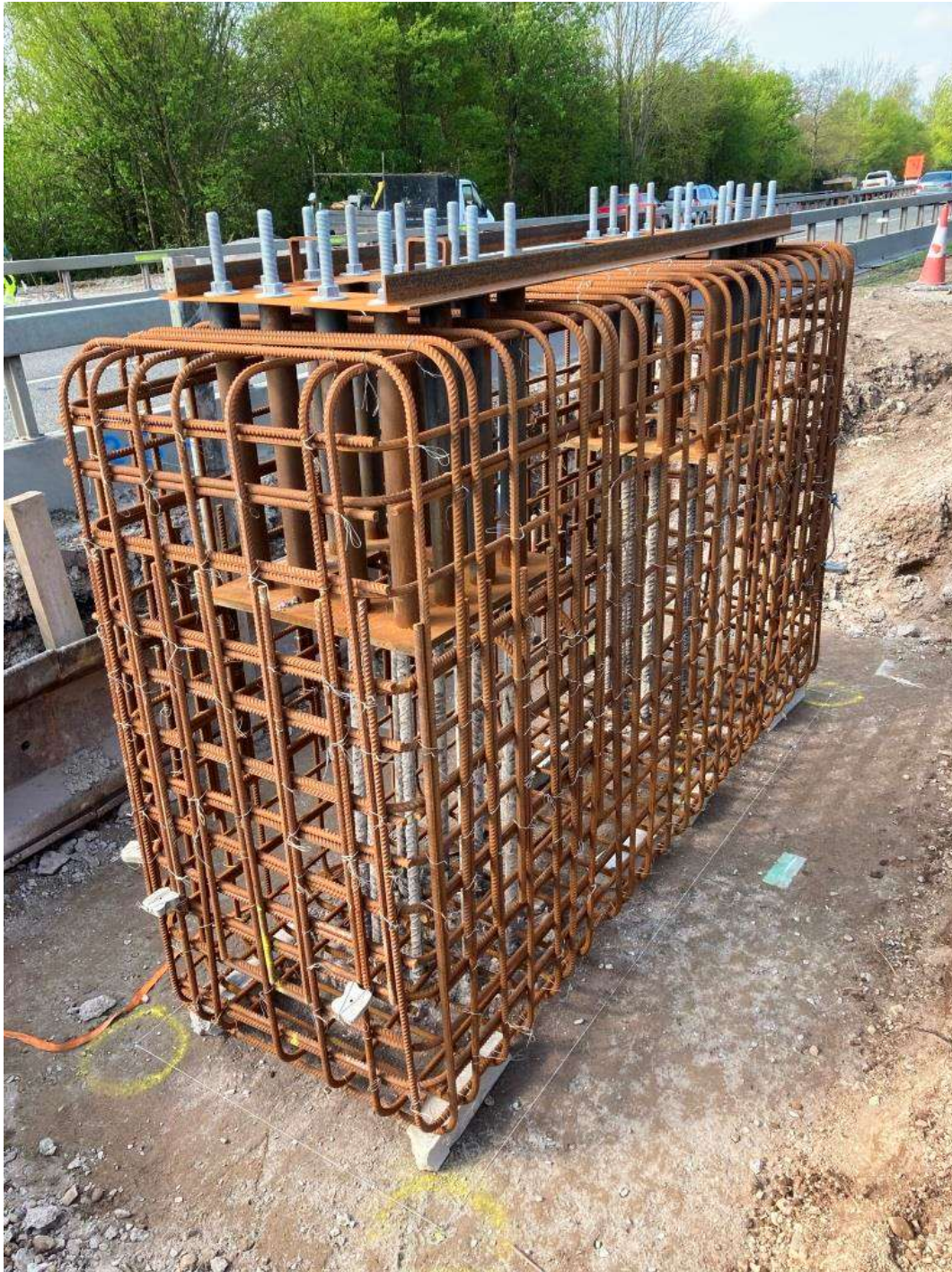
Piled portal gantry foundation with steel fixed and holding down bolts in place ready to receive the formwork
