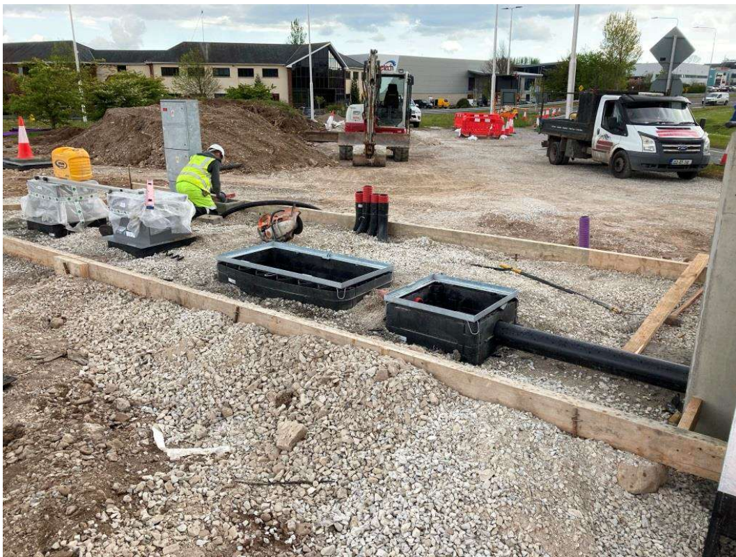
Preparation of the concrete plinth around the ITS equipment on the N25 eastbound near the Little Island Interchange.
