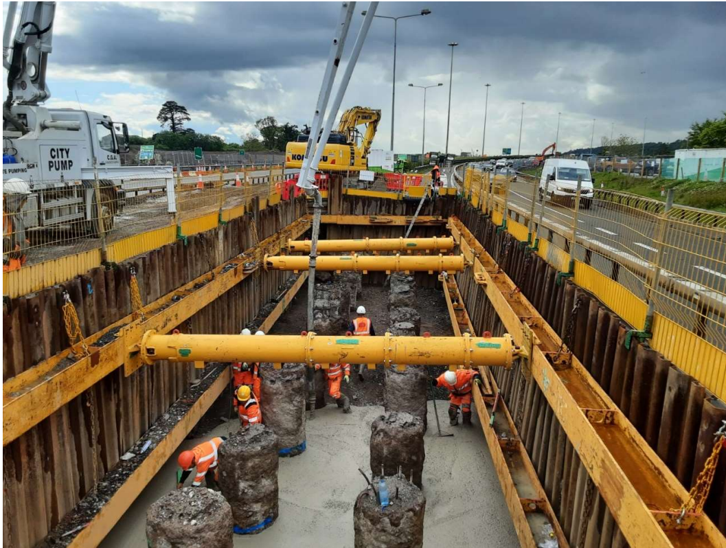
Concrete blinding being installed in the ST01 cofferdam in the existing N25 central median.
