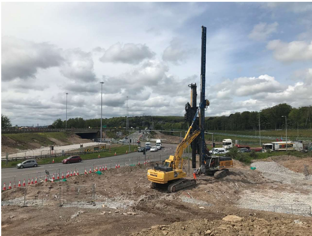
Installation of prefabricated vertical drains ongoing.
