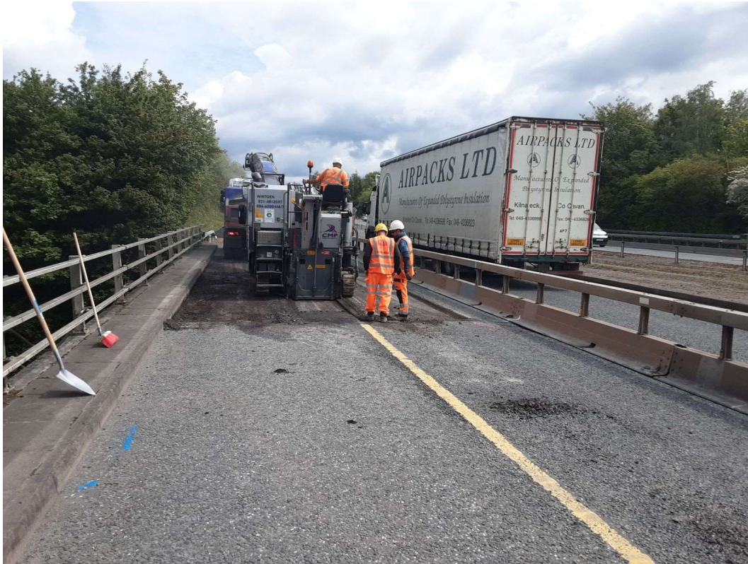
Road planing works at ST10 on the M8 northbound underway.
