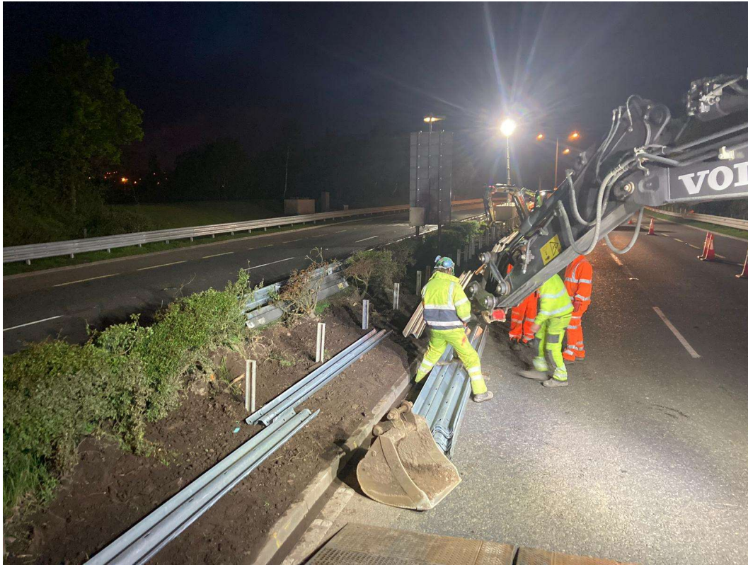
Safety barrier installation on the N40 during night time lane closures.
