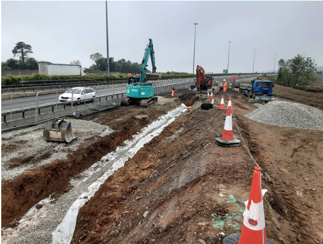
Drainage Installation ongoing alongside the N25 eastbound.
