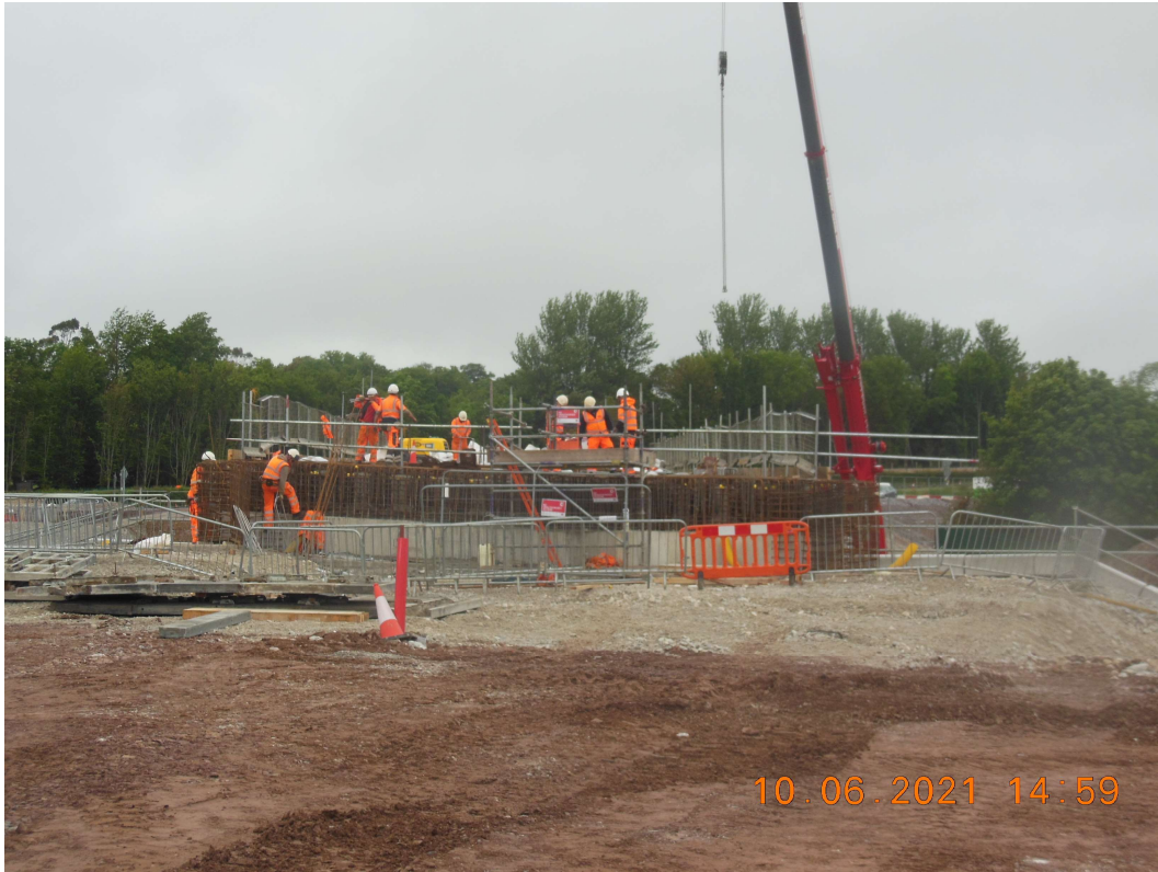
Steel fixing works ongoing at ST09.
