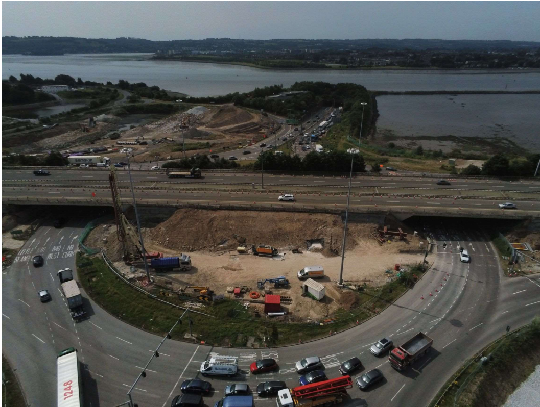
Soil nailing and piling works ongoing at the Dunkettle Interchange Roundabout.
