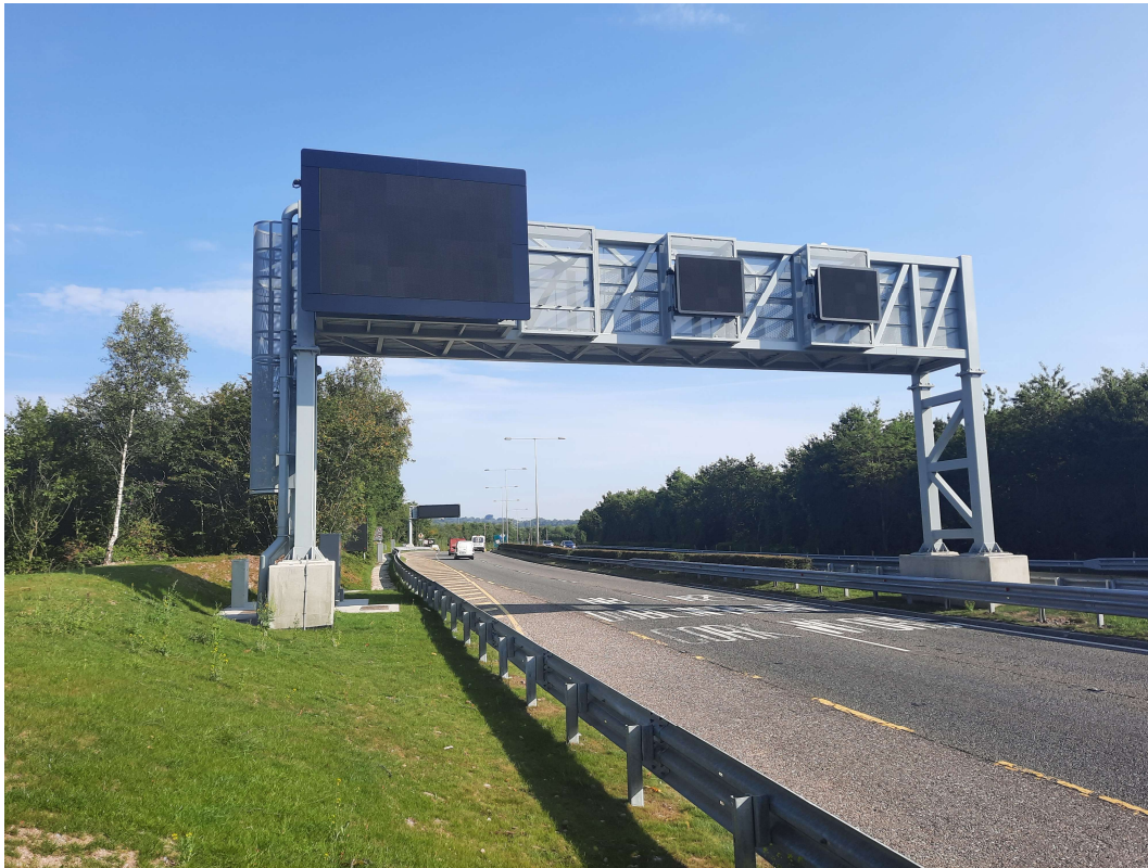
Structural steel portal gantry on the N40 eastbound with an Enhanced Message Sign and Lane Control Signs in place.
