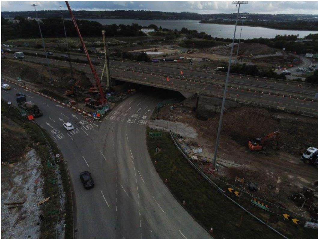
Ongoing piling works for ST07 at the eastern side of the Dunkettle Interchange Roundabout.
