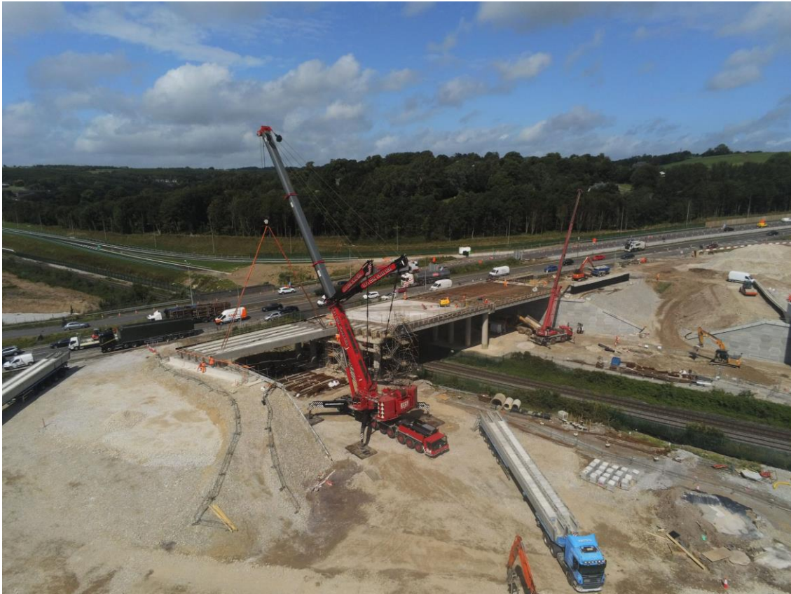
Bridge beams for the ST08 southern deck being installed parallel to the live M8 southbound.
