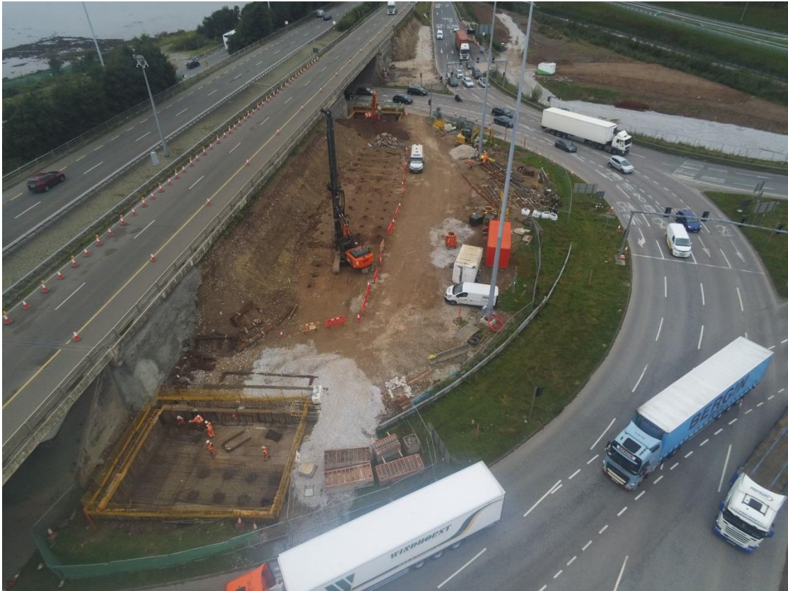
CMC works being undertaken within the central island between the works for ST06 & ST07.
