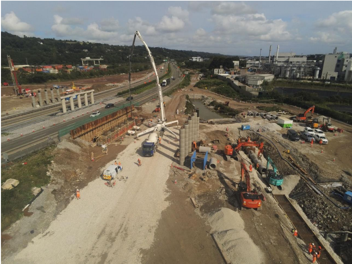
Installation of Culvert 07 ongoing just south of ST01 as the southern central pier pile cap is being poured.
