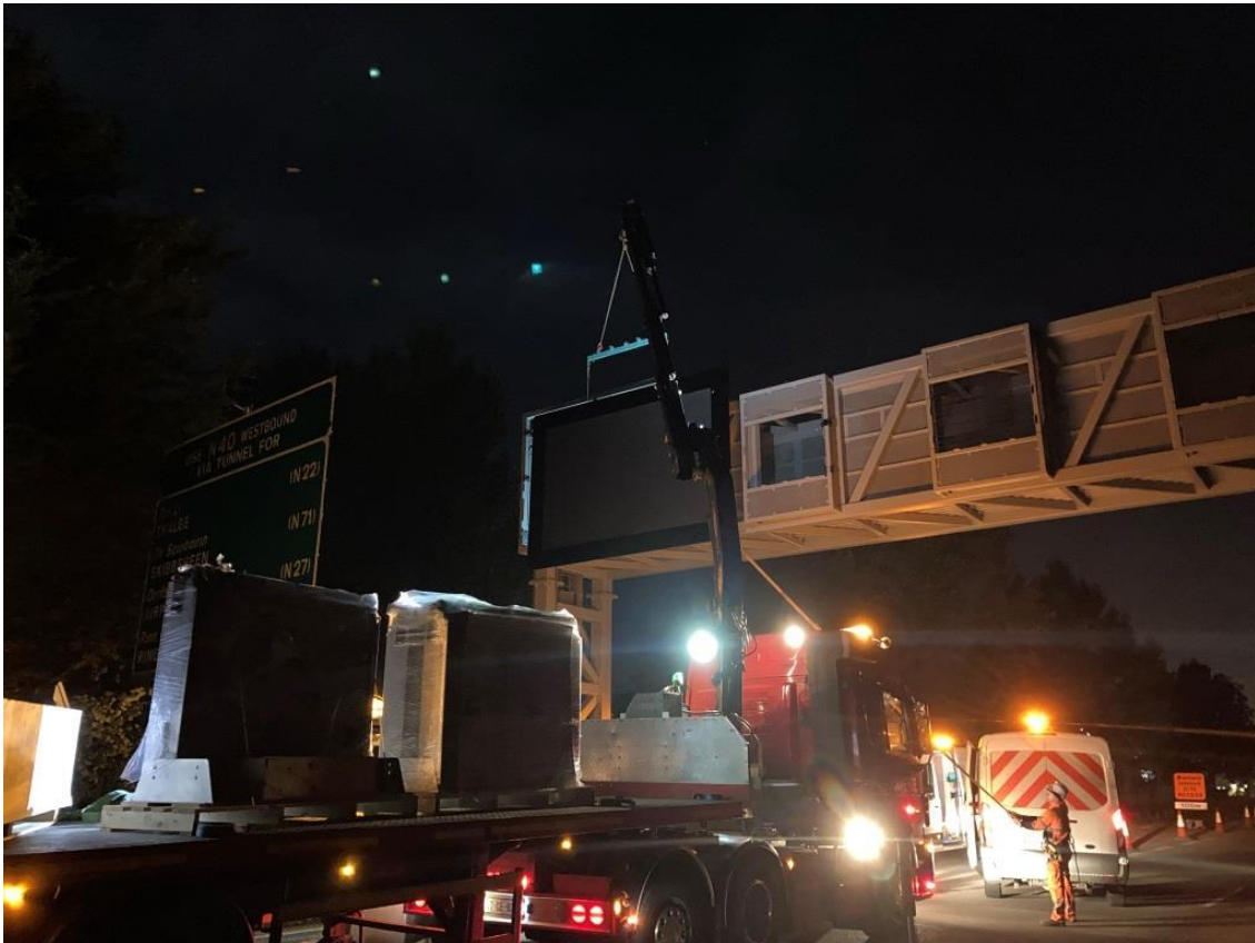
Enhanced Message and Lane Control signs being installed on the N25 Westbound.
