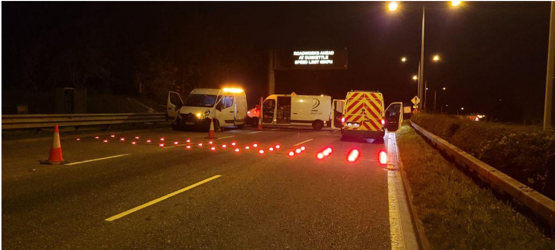
Warning road studs being tested during installation on the N40
