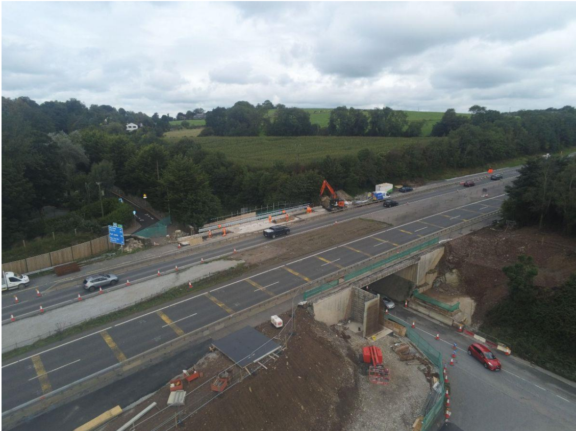
Parapet upgrade works nearing completion at the M8 Northbound
