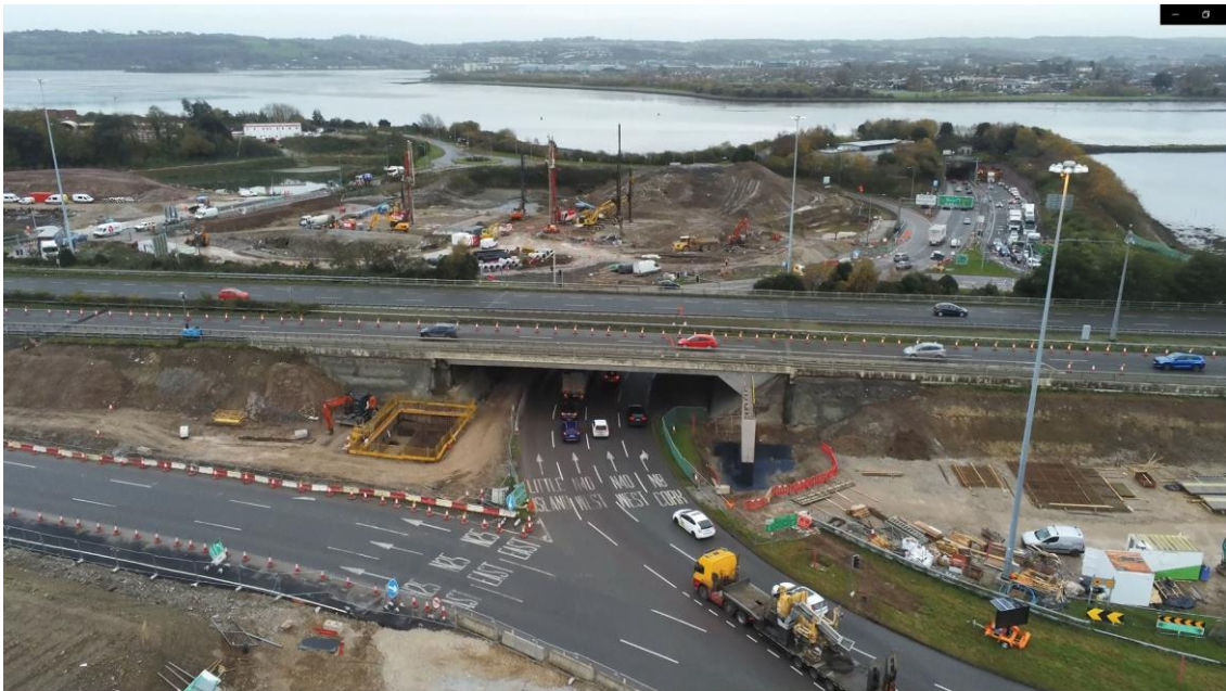
CMC ground improvement works ongoing for Link C in the area South of the N25 with ST07 in the foreground also.
