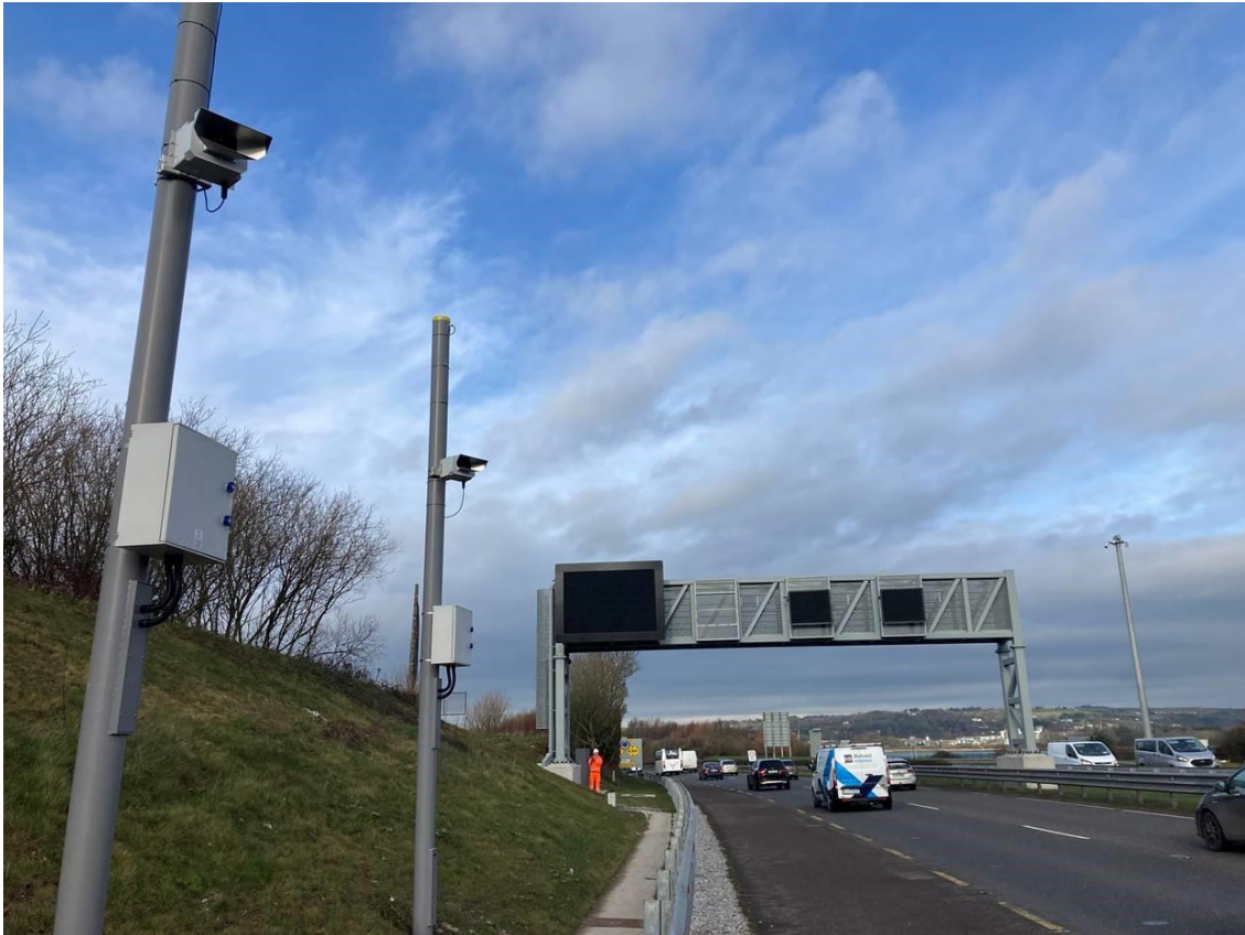
ITS on N40 Approach to Tunnel, including newly installed Over-Height Vehicle Detectors in foreground.
