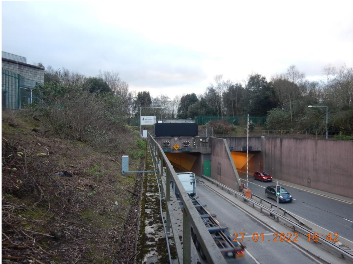
Recently installed VMS overhead the entrance to the southbound bore of the Jack Lynch Tunnel.
