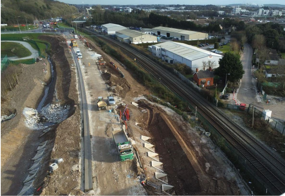
Installation of the concrete surface water channel ongoing at Link T1.
