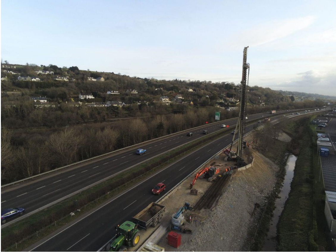
Piling works ongoing alongside the N25 westbound.
