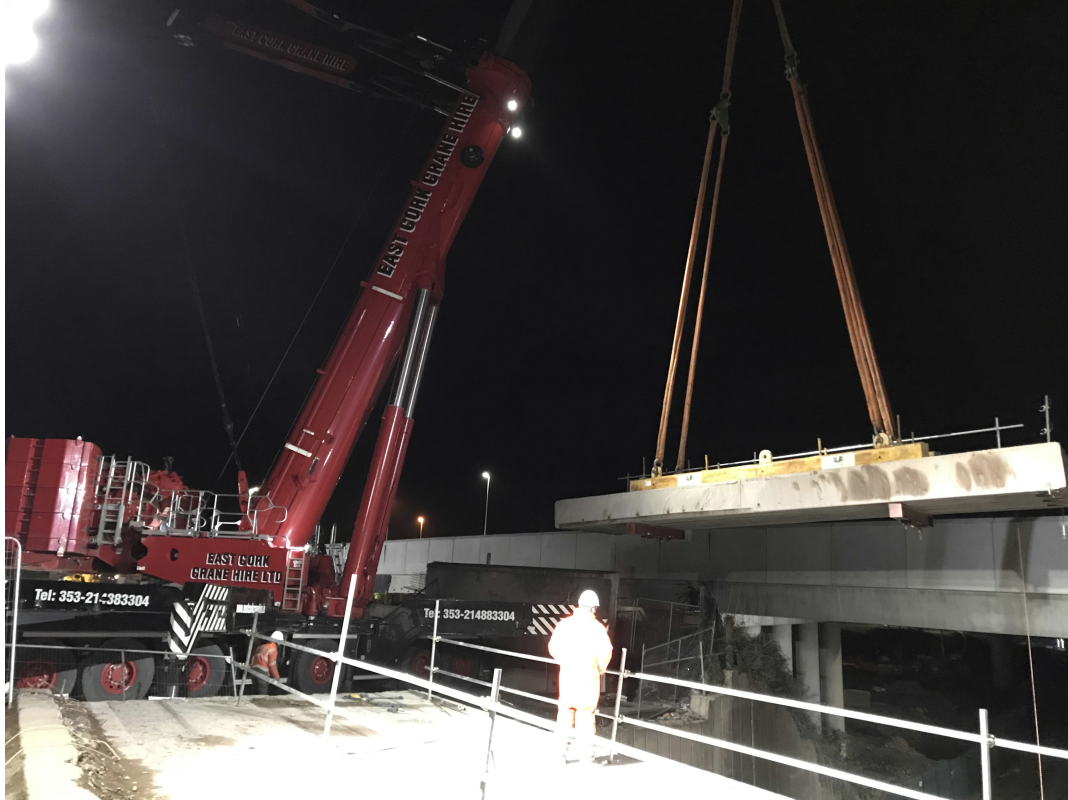
Removal of the existing railway bridge deck in sections ongoing at night.
