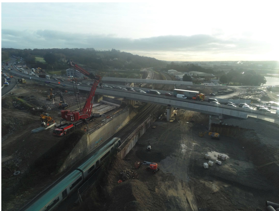
The existing railway bridge deck removed alongside the recently constructed Structure St08.
