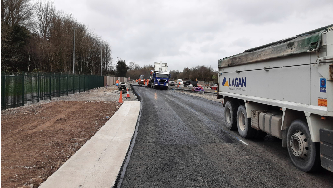
Pavement tie in works being completed for the Link U tie in with the M8 northbound.
