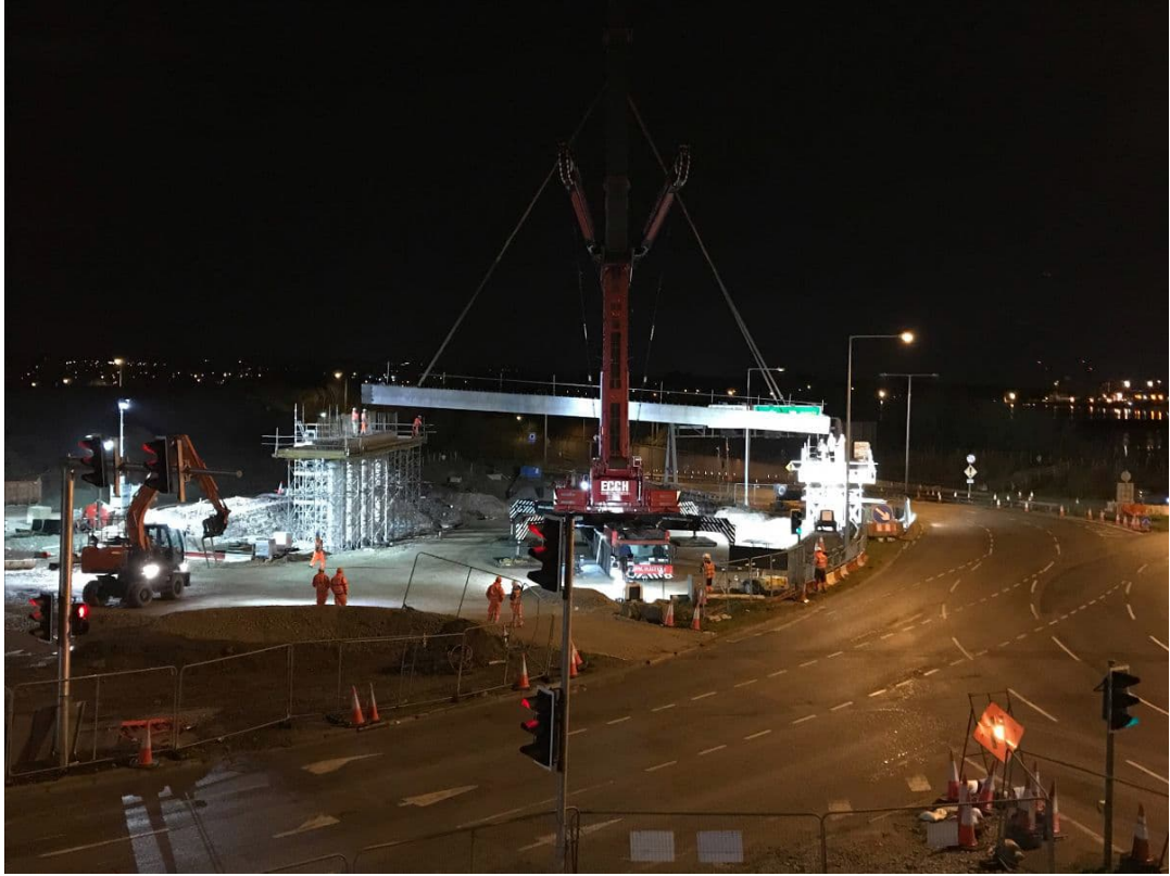
Installation of the beams at Structure St05 at night time alongside the Dunkettle Interchange Roundabout.
