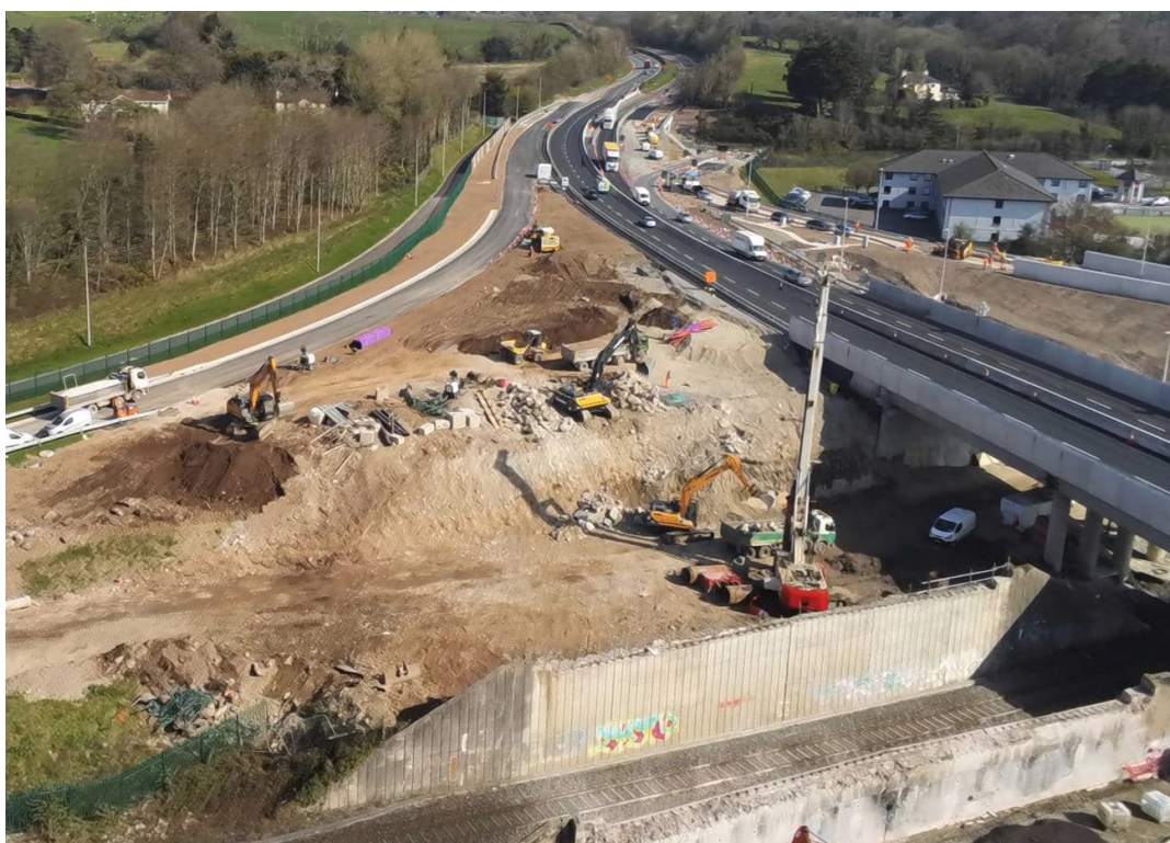
Structure St08 piling works ongoing alongside the M8 northbound.
