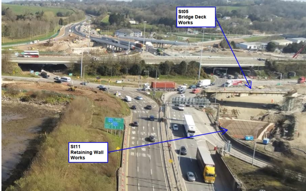
Steel fixing works being progressed at Structures St05 & St11.
