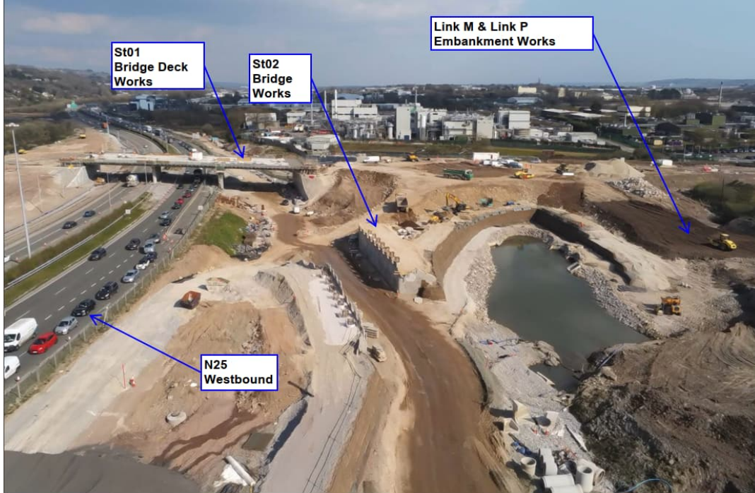
Completion of the earthworks embankments for Link M & Link P.
