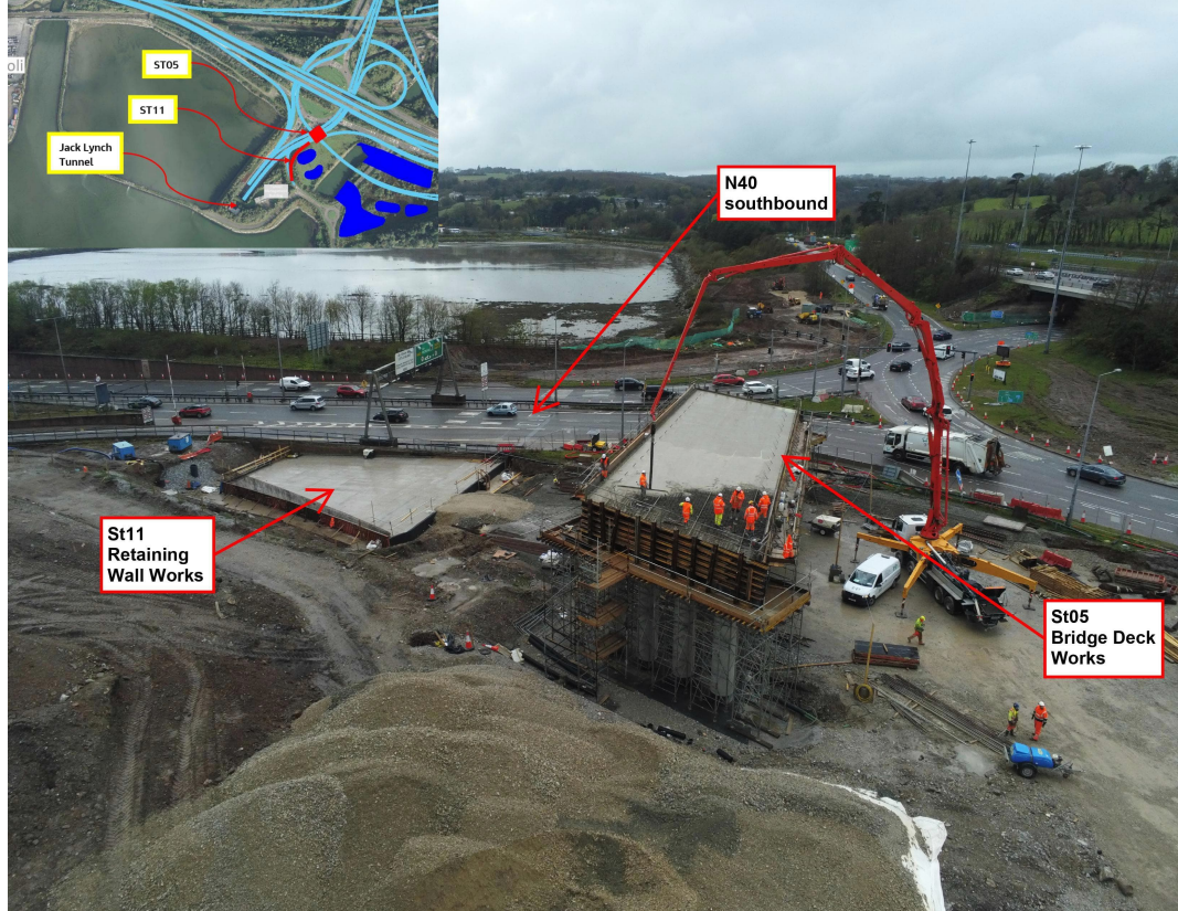
St05 bridge deck pour ongoing alongside the N40 southbound.
