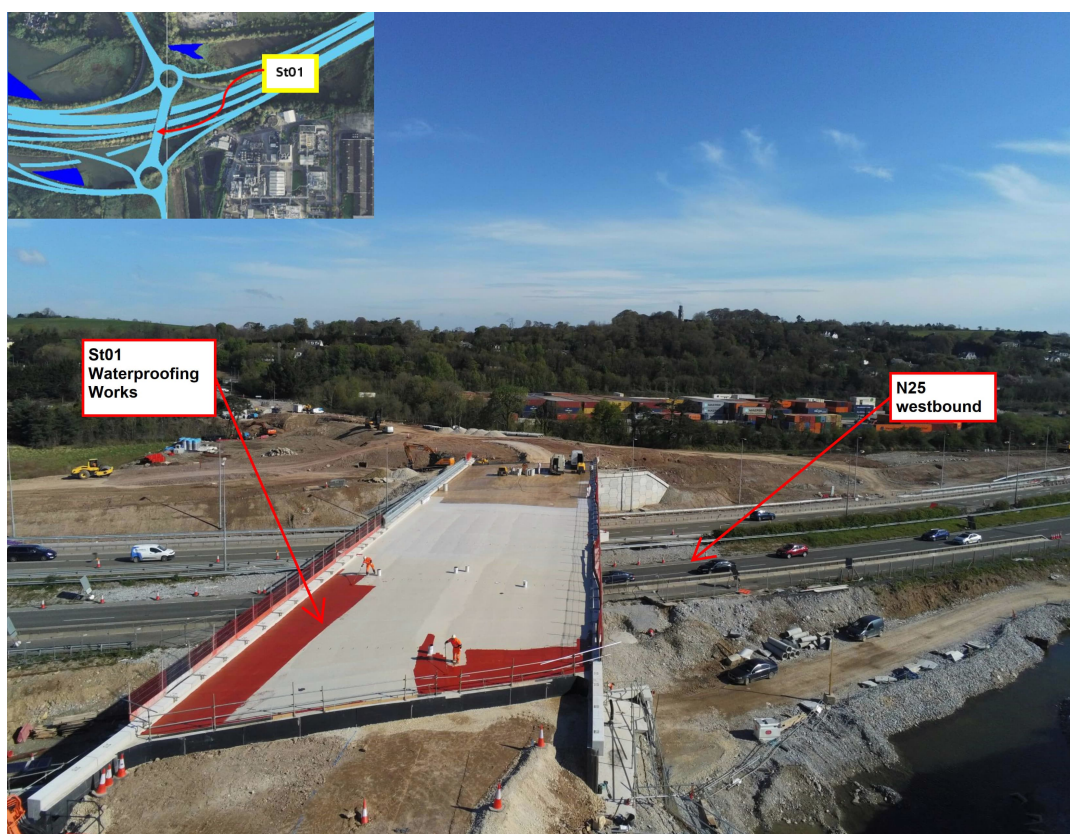
Waterproofing works at St01 over the N25
