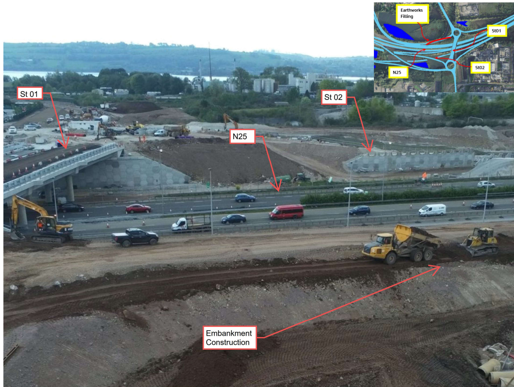
Embankment construction ongoing north of Structure St01.
