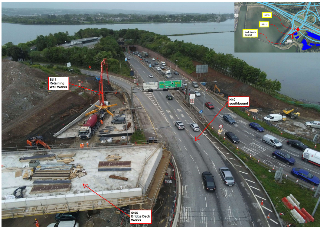
Concrete being pumped into position alongside the N40 southbound.
