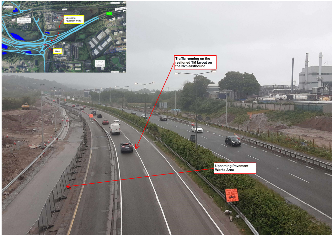
Realigned traffic management layout on the N25 eastbound alongside Structure St01.
