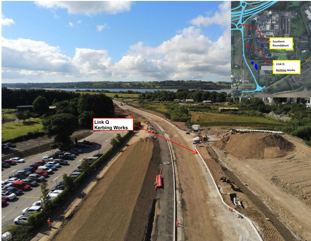
Kerb installation completed at Link Q.
