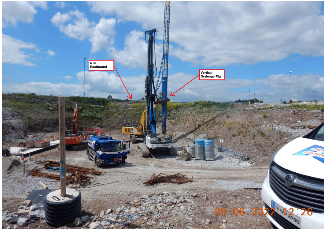
Vertical drainage rig in operation at Link F.
