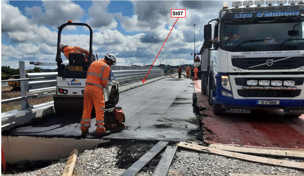
Pavement materials being placed at Structure St07 alongside the N25 eastbound.
