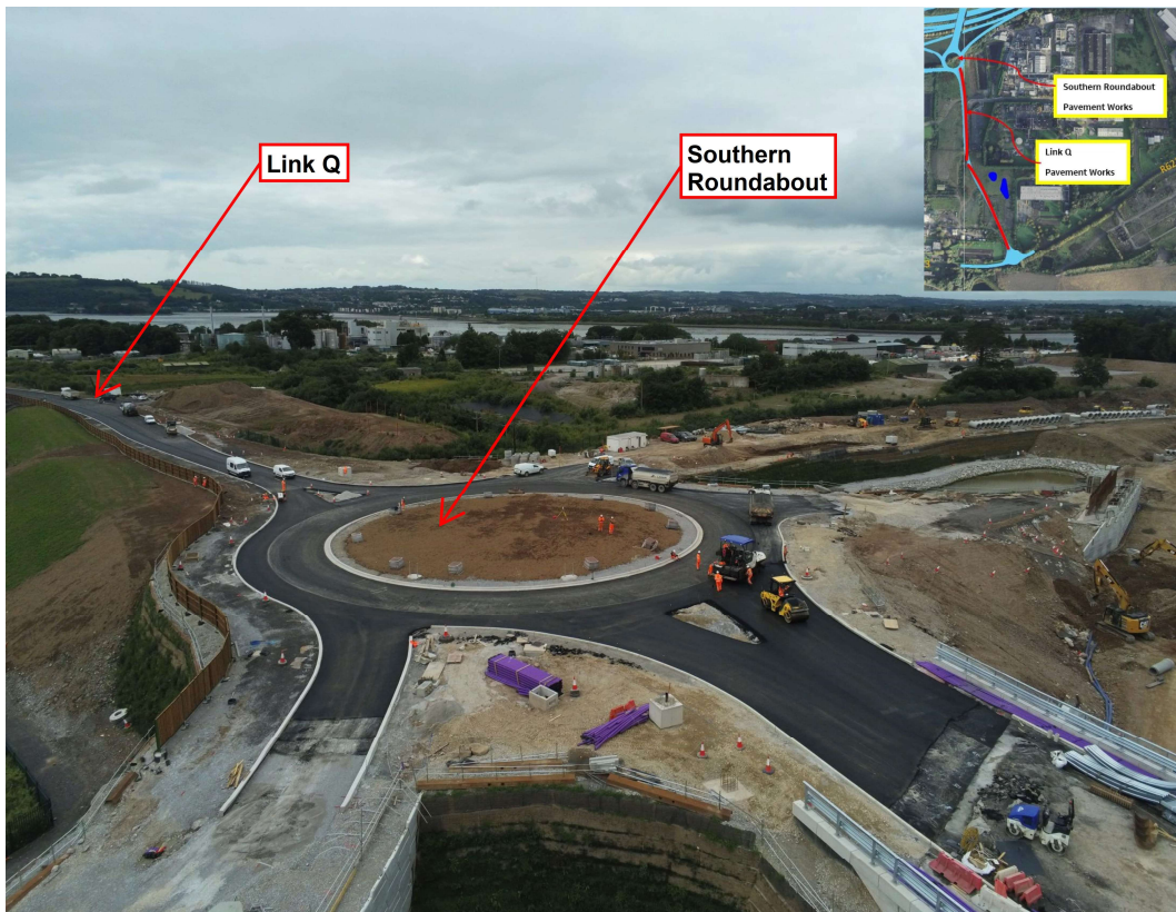
Pavement works ongoing at the Southern Roundabout / Link Q area.
