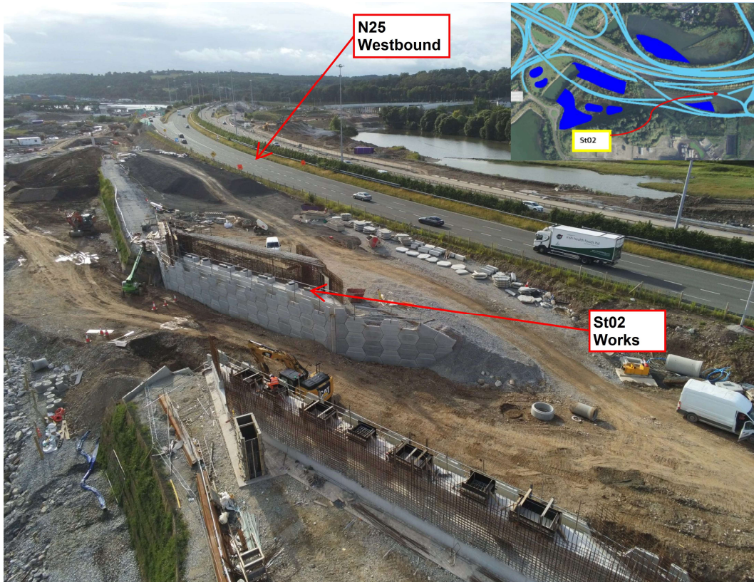
St02 works ongoing alongside the N25 westbound.
