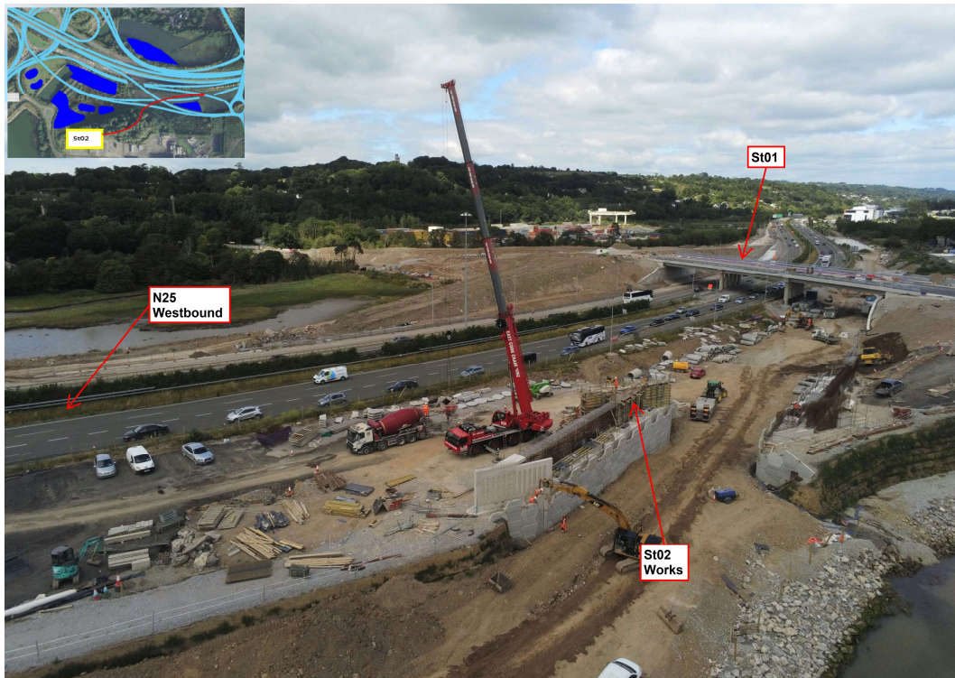
Wing walls being poured at Structure St02.
