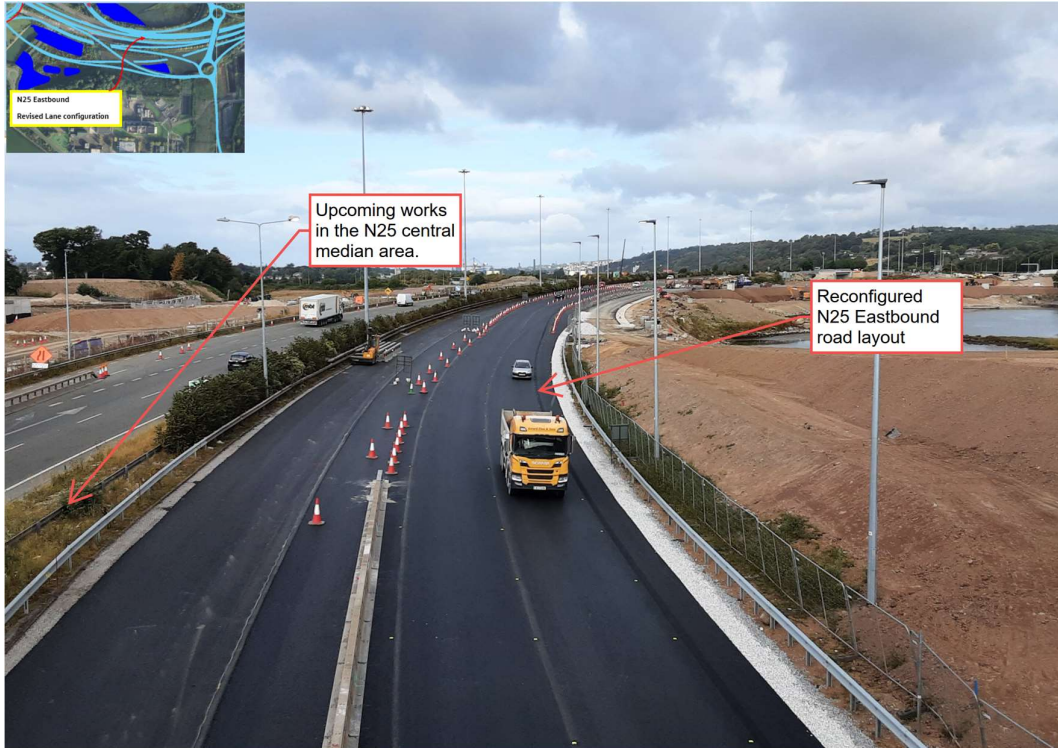
Current lane configuration on the N25 eastbound.
