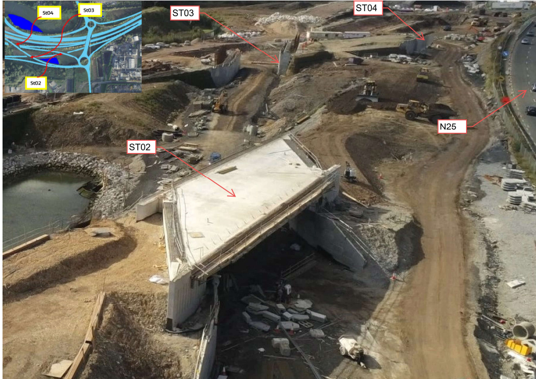
Works continuing at Structures St02, St03 & St04 alongside the N25 westbound.
