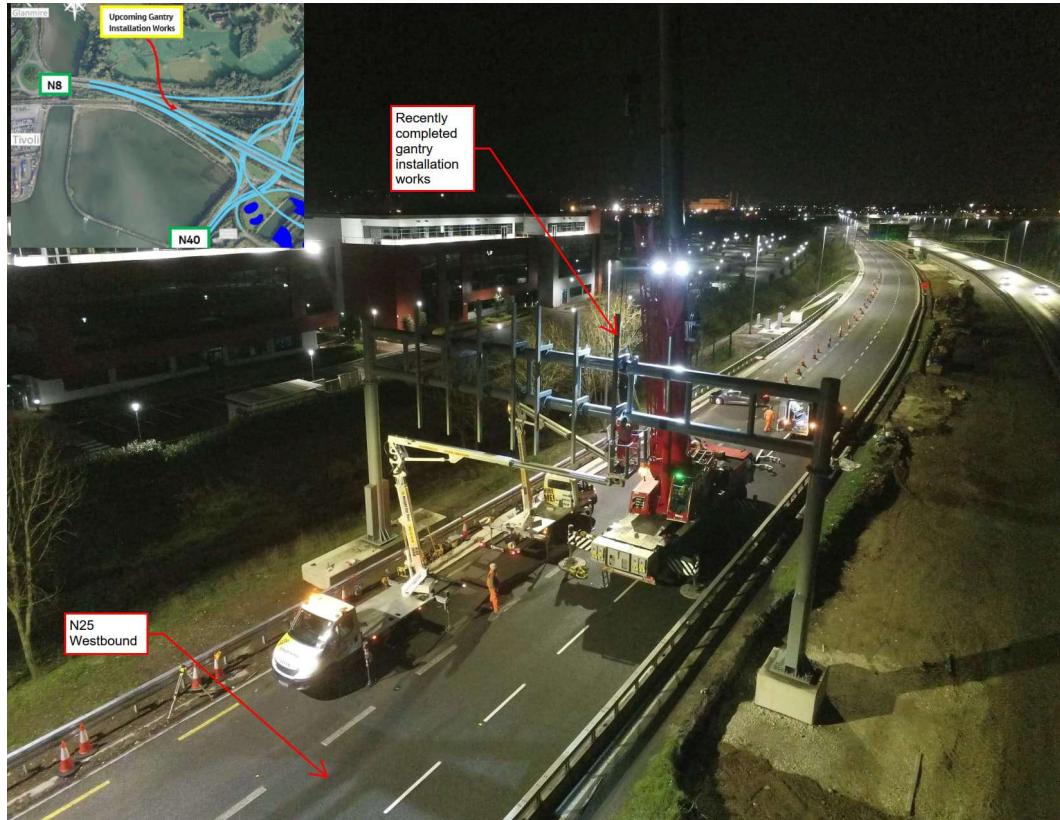
Gantry signage installation works ongoing on the N25 under night-time working.
