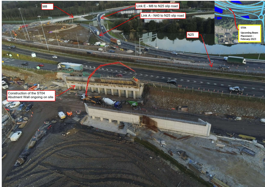
Completion of a further concrete pour at Structure St04 alongside the N25 Westbound.
