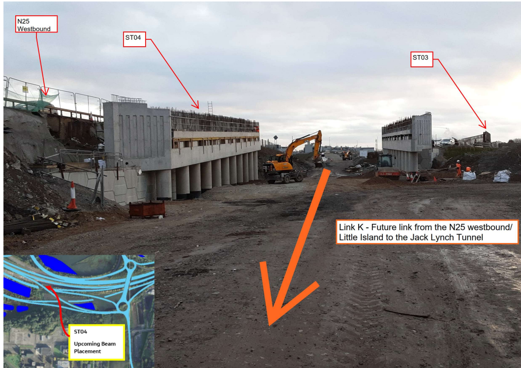
Structure ST04 alongside the N25 Westbound ready for the installation of beams.
