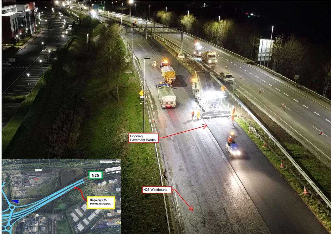
Pavement works being undertaken at night on the N25 westbound.
