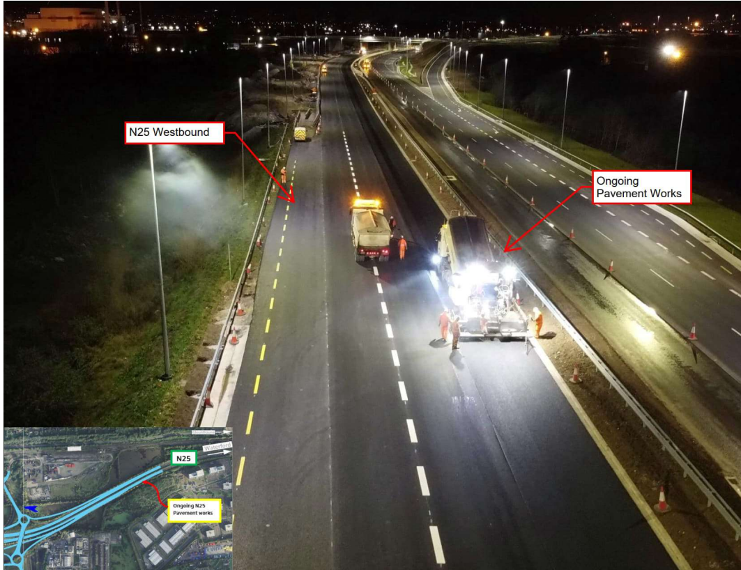
Pavement works being undertaken at night on the N25 Westbound.
