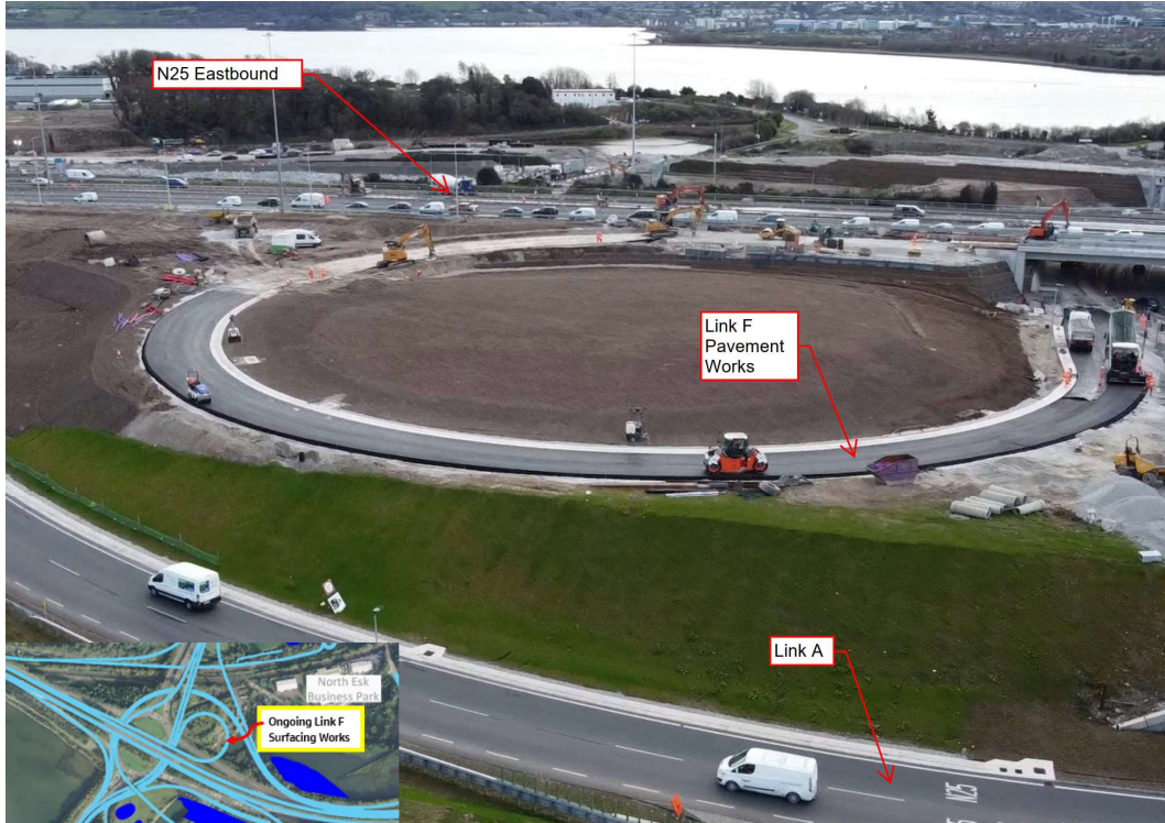
Surfacing works being undertaken at Link F.
