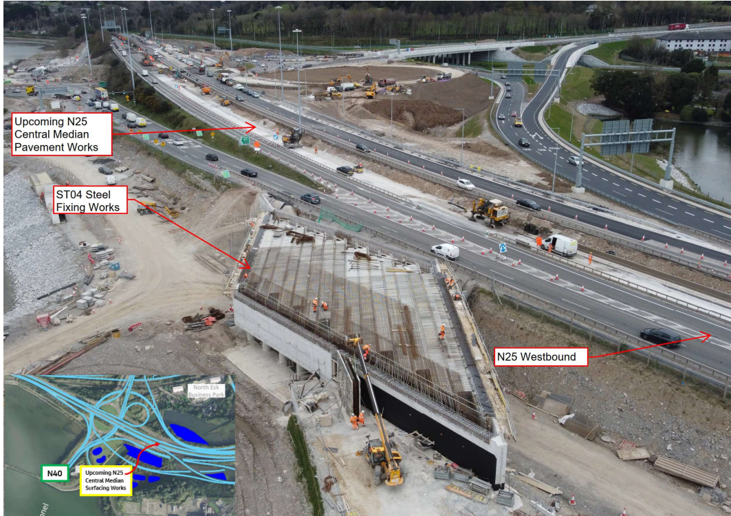
Preparatory works ongoing for the upcoming N25 central median pavement.
