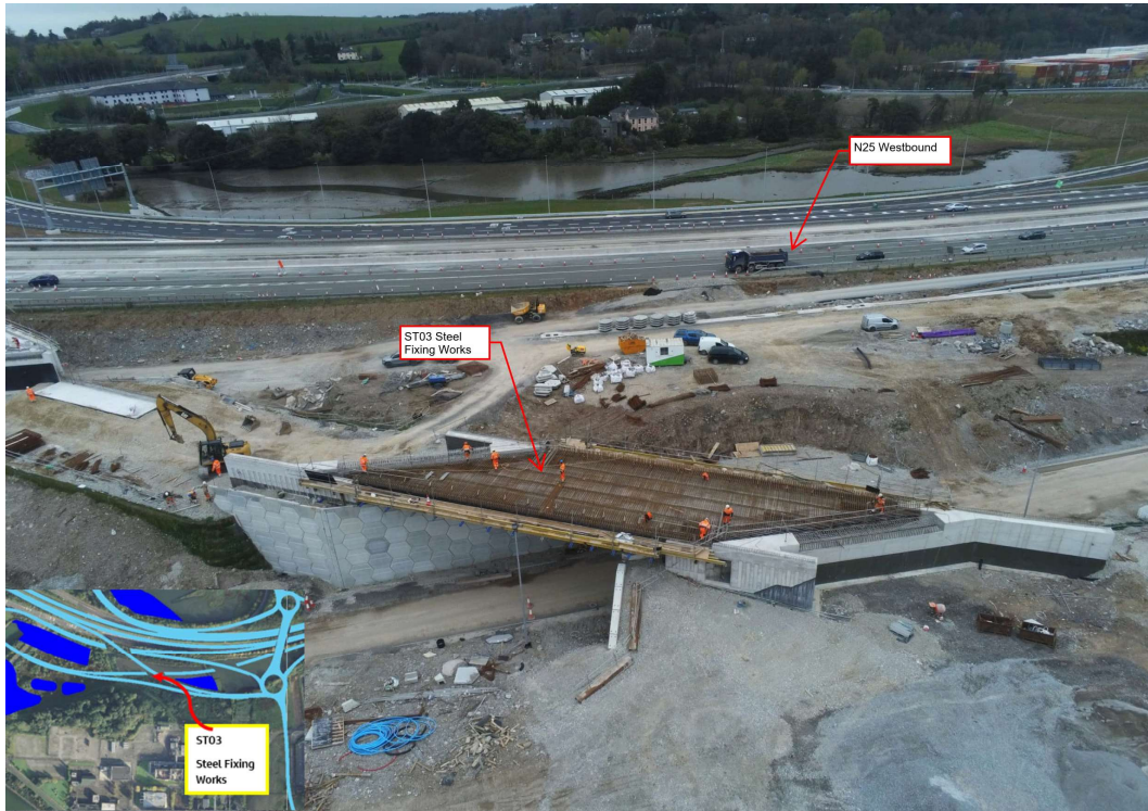
Steel Fixing Works ongoing at Structure ST03.
