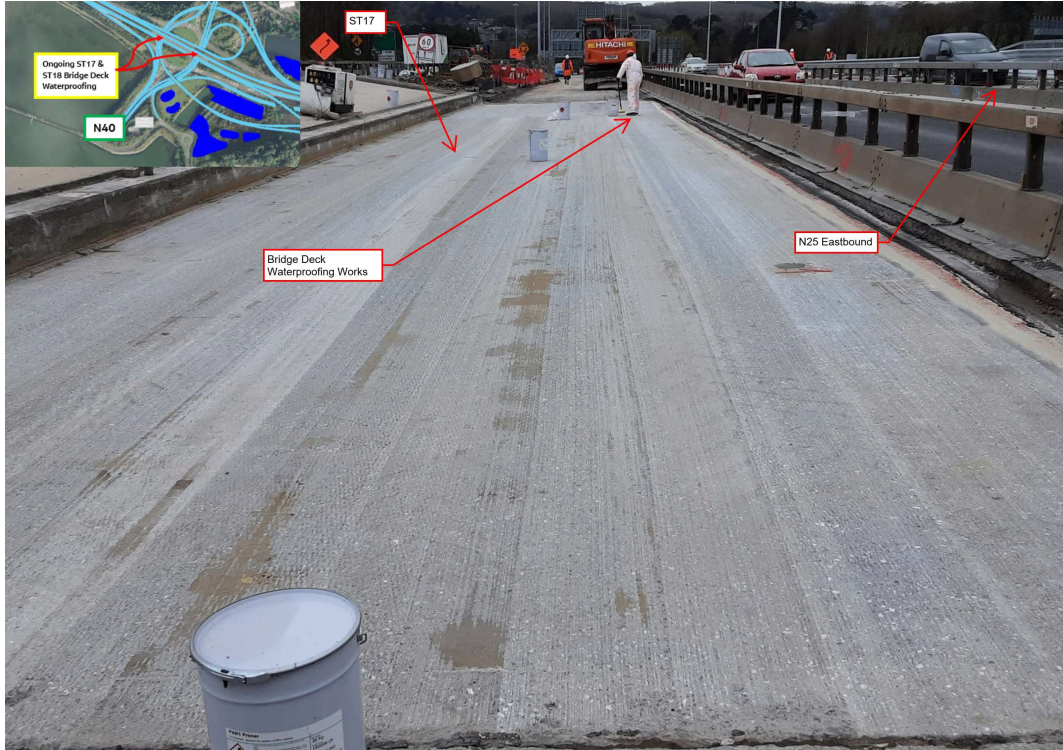
ST17 Bridge Deck being prepared to receive waterproofing.
