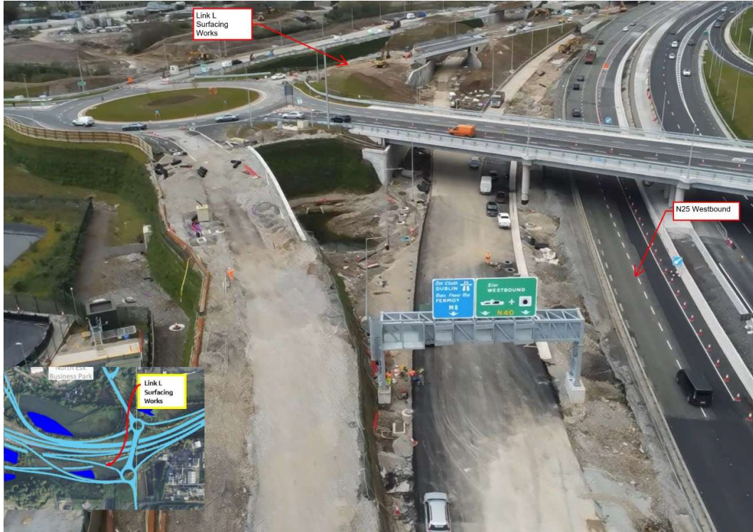
Upcoming surfacing works alongside the N25 westbound.
