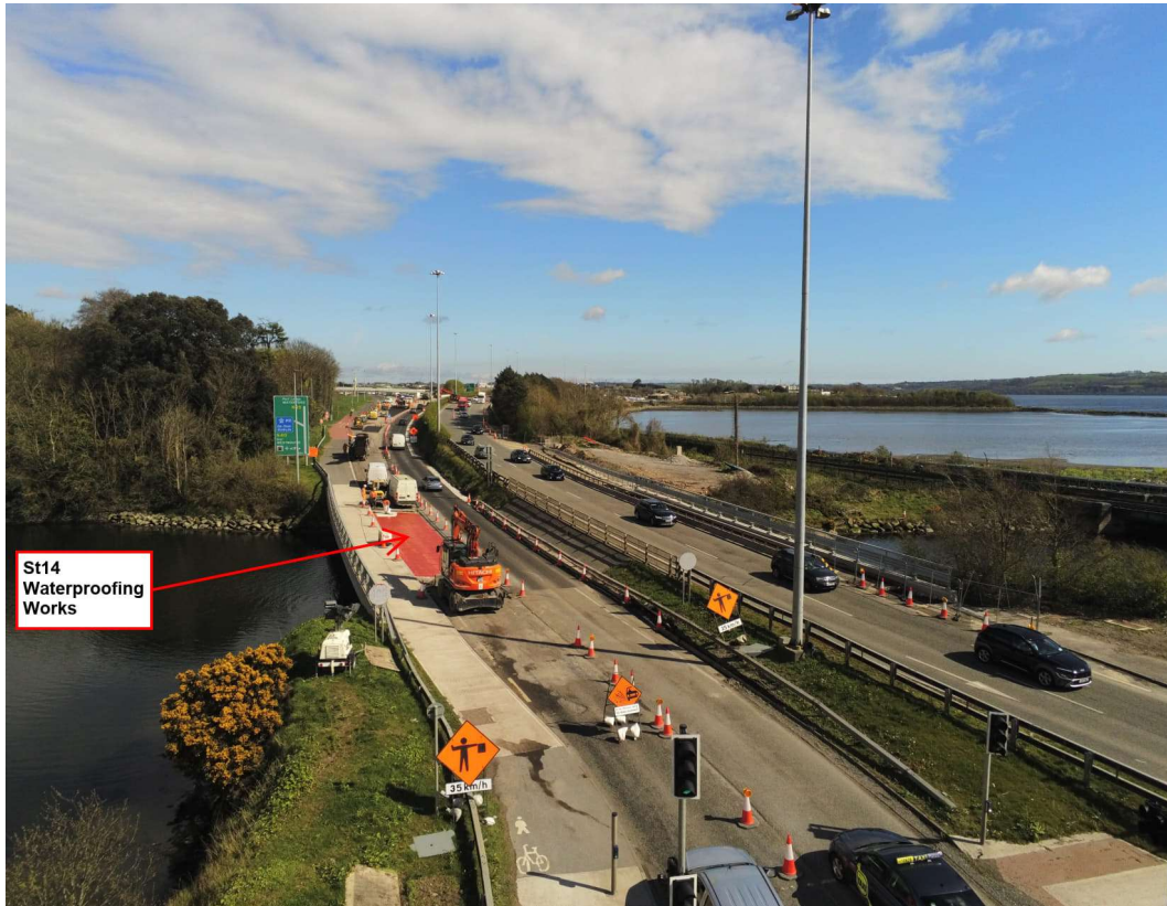
Waterproofing works being completed previously at ST14 under the N25 Eastbound.
