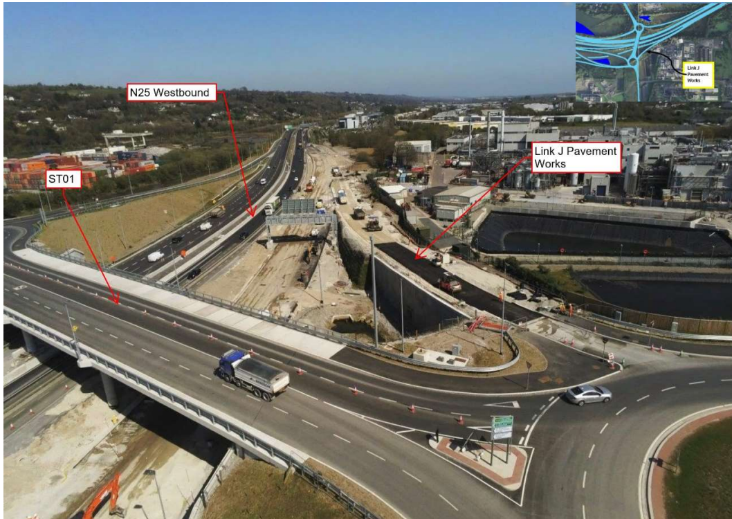
Pavement works ongoing at Link J.
