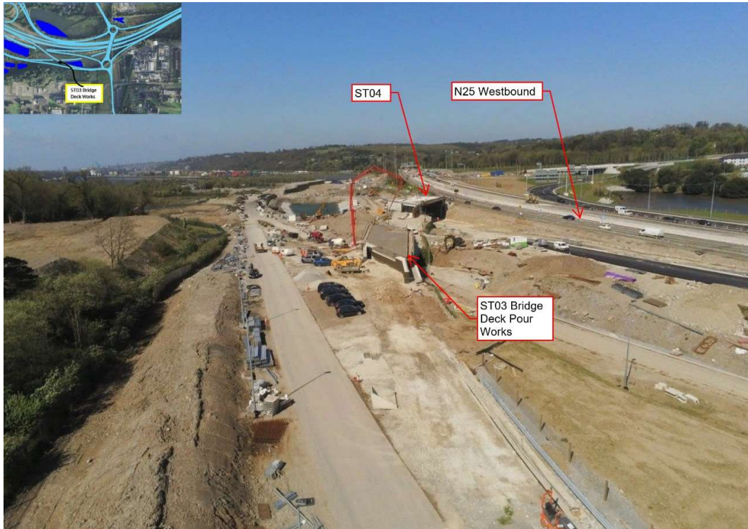
Concreting works ongoing at Structure ST03.
