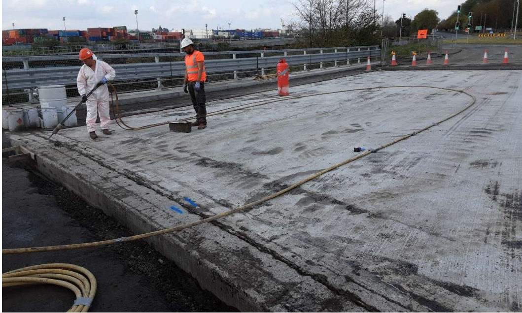
Bridge Deck Waterproofing works at Structure ST14.
